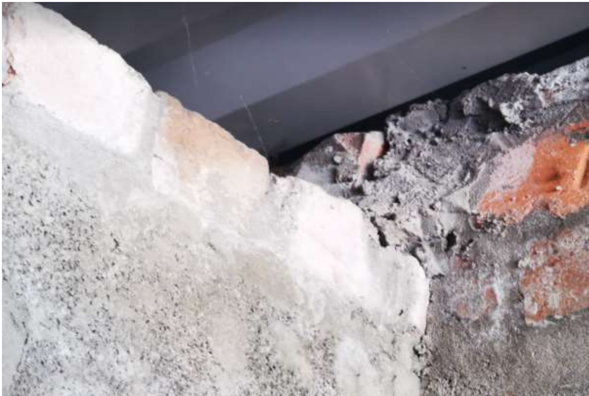
Plate 2- Gaps at wall plate level with no light ingress'
