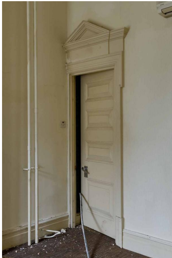
Figure 19. Doorcase and panel door to store in Room 4.
