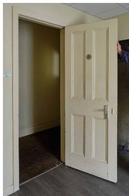
Figure 24. Panel door to ladies toilet.
