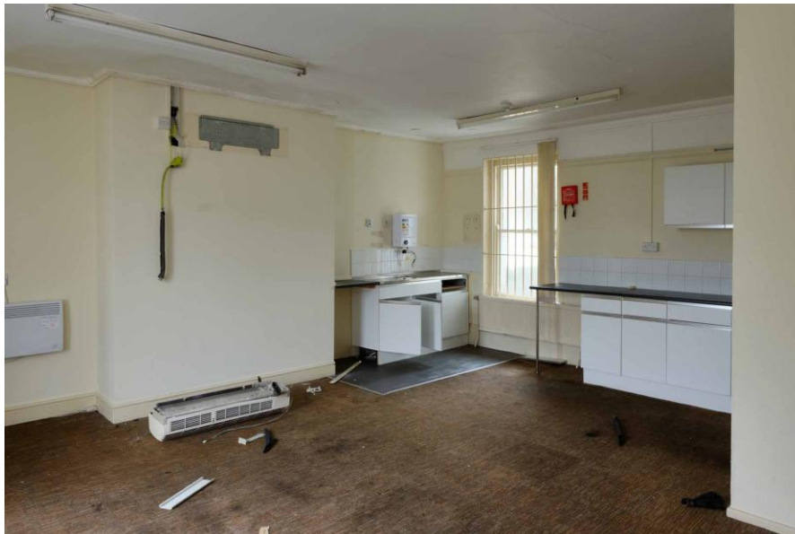
Figure 23. Room 6, with blocked fireplace.
