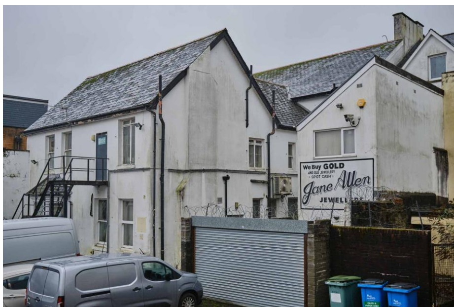
Figure 9. Rear of the building, showing the lower link to the parallel rear range.
