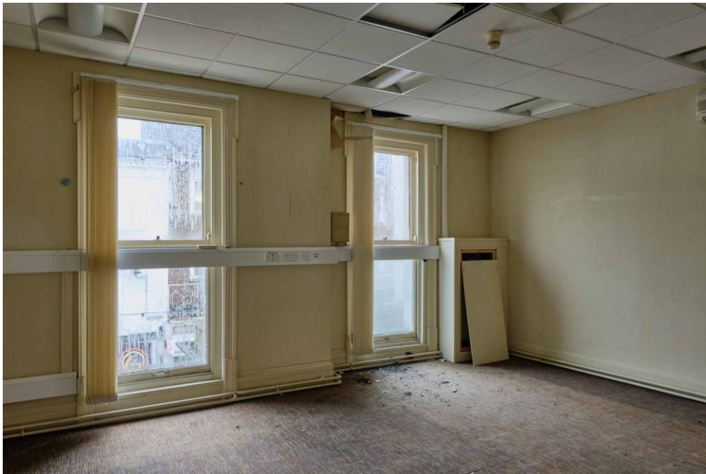
Figure 20. Architraves to windows in Room 1.
