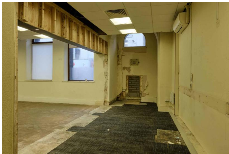
Figure 12. View to the blocked former entrance, with evidence of a former corridor separate from the banking hall.
