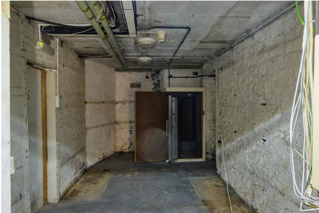
Figure 27. Basement, with small modern safe, and dividing wall on the right, probably pre-dating the first bank on the plot.
