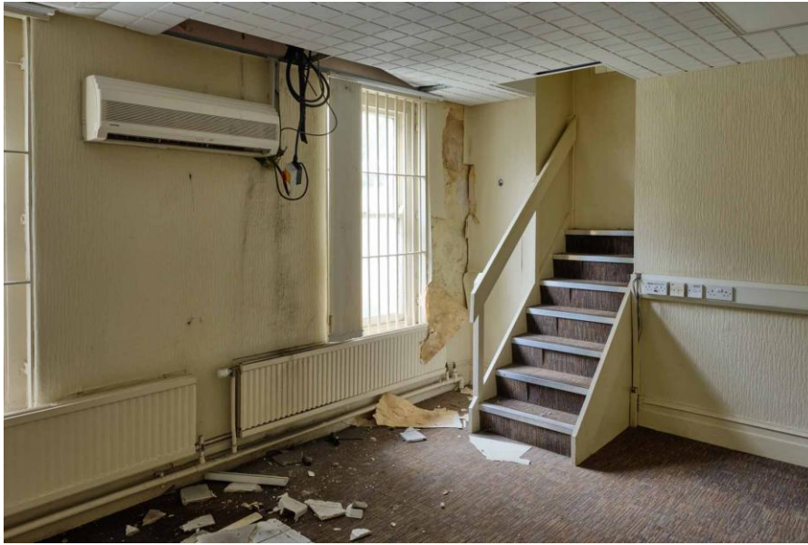
Figure 22. Modern steps in Room 5, and barred window.
