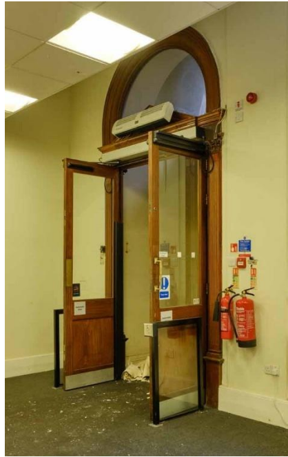
Figure 13. Inner doorway of main entrance.
