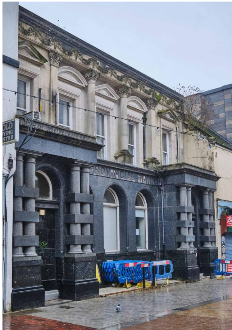
Figure 5. Entrance front on High Street.
