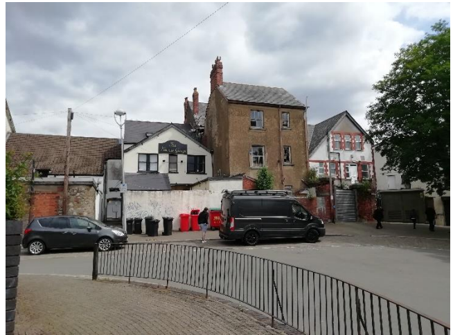
Figure 9 - Buildings nearby (to north) with PRFs
