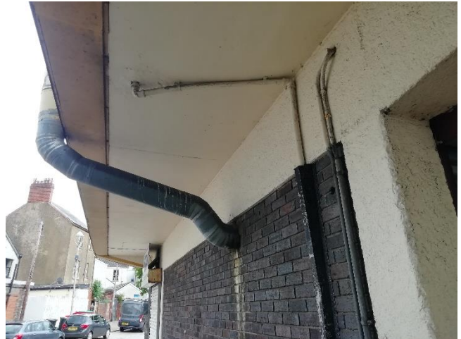
Figure 3 – Typical overhang tightly sealed from below
