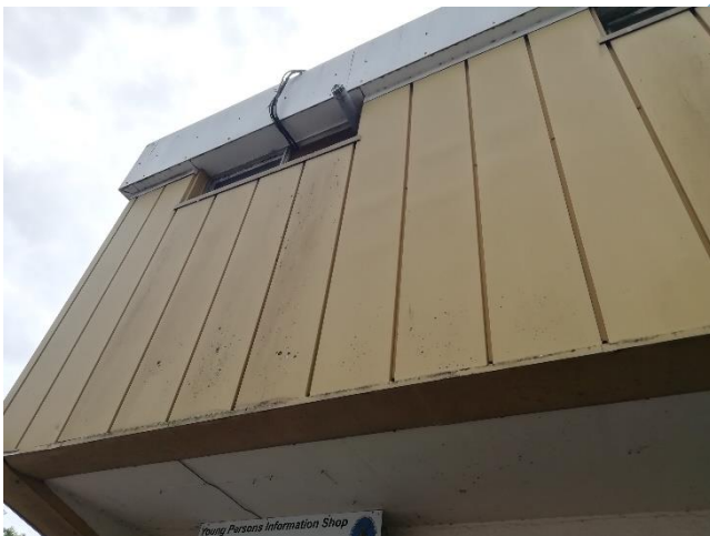
Figure 4 – Cladding of main section
