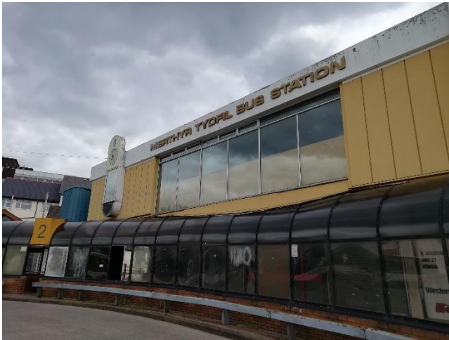
Figure 8 – View of western elevation
