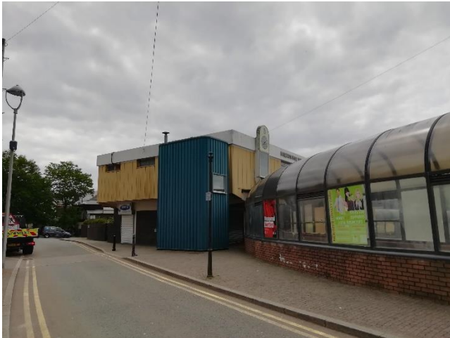
Figure 2 – View along northern elevation, view to east
