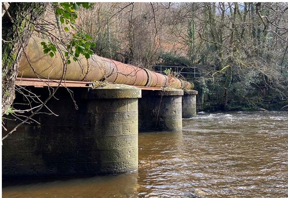
Figure 1-2: Existing Bridge Structure
