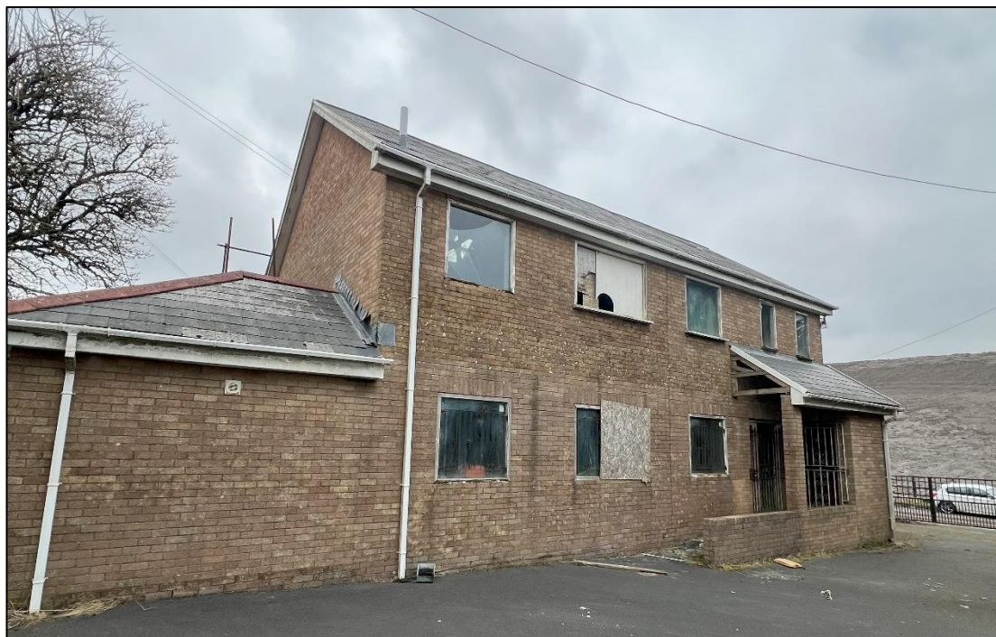
Figure 3.3 One of the existing buildings within the site.
