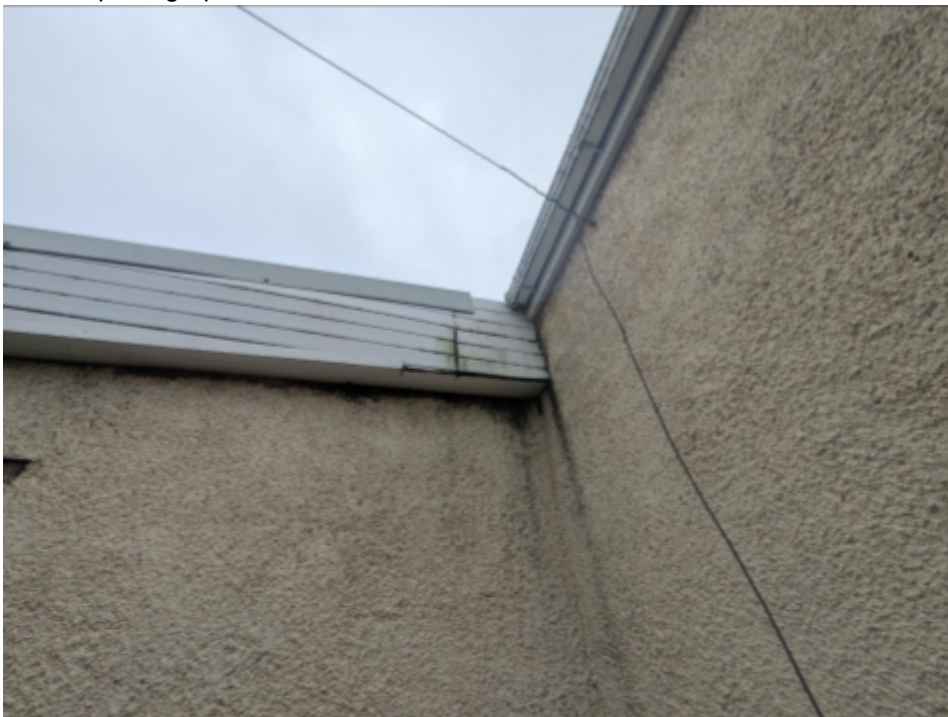
Plate 2- photograph of sealed fascias and soffits
