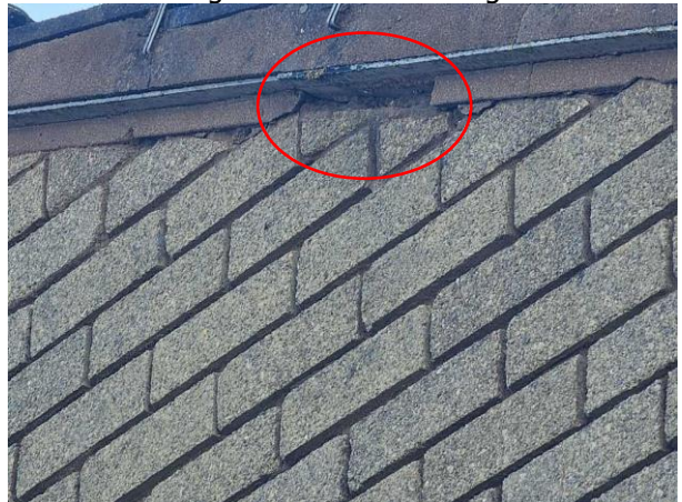
Photo 6: Missing mortar on western gable
