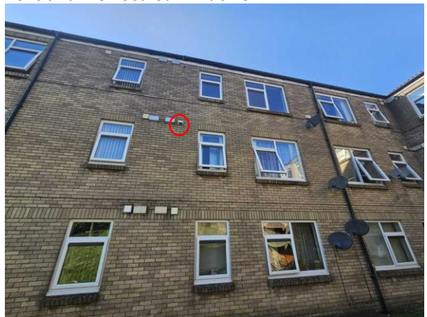
Photo 6: Missing mortar on western gable
