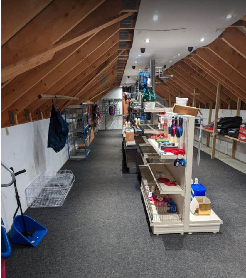
Plate 7- photograph of loft over north eastern end of building
