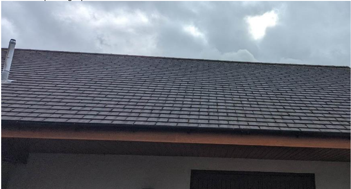
Plate 8- example of tightly fitted roof
