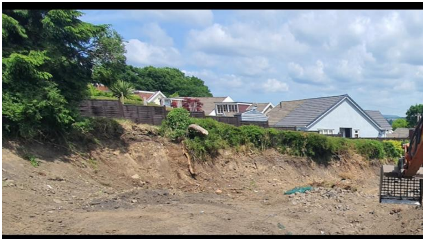
Figure 1 - Retained northern boundary hedge/bush on the elevated boundary above the development platform / proposed dwelling FFL; retaining wall to be constructed below.
