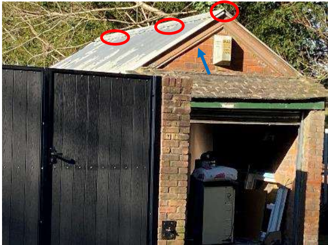
Photo 9: Southern and eastern elevation Showing gaps between ridge flashing and corrugated metal roof ( red circles refer) and gaps at barge board at the gable end ( blue arrow refers)
