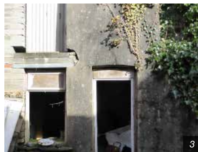
3. Bowens Court - Sand Cement render meeting more modern blockwork wall, vegetation covering large parts of elevation
