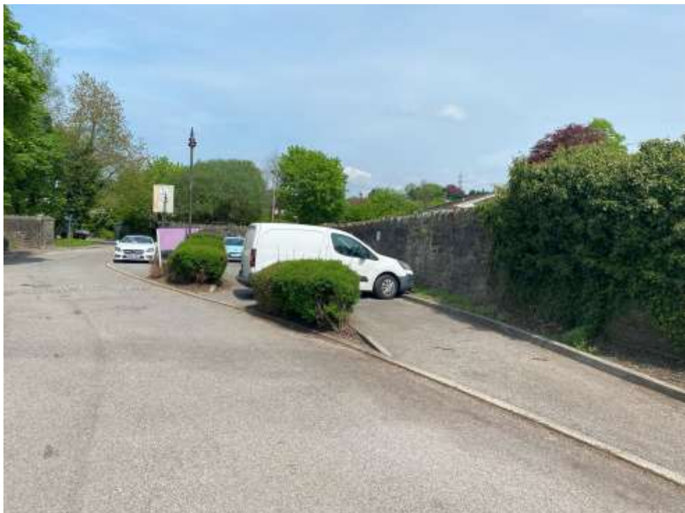
Plate 10 – Stone boundary wall to the northeast corner of the Site.
