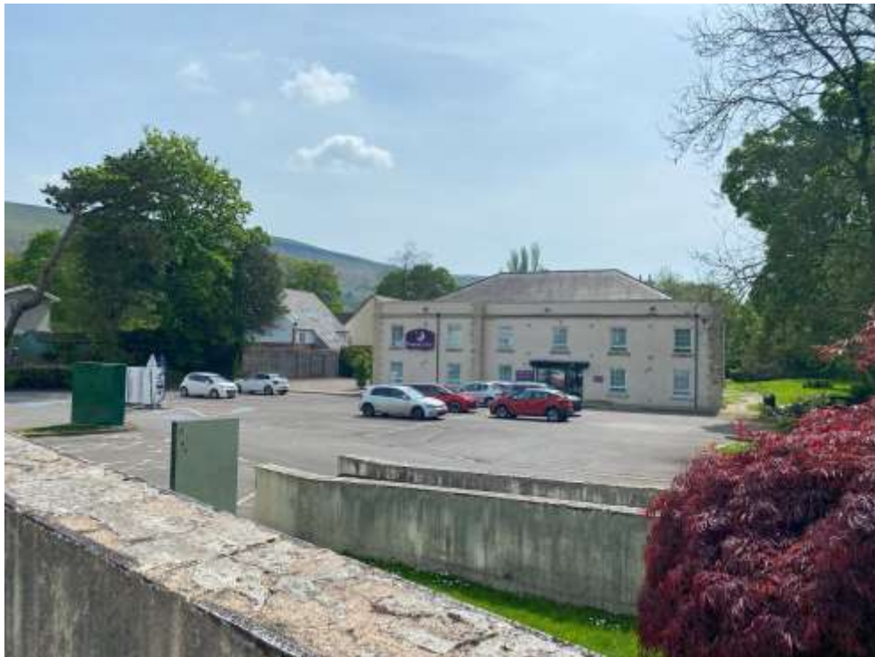
Plate 6 – North elevation of the extant hotel block viewed from the southern extent of the restaurant garden area.
