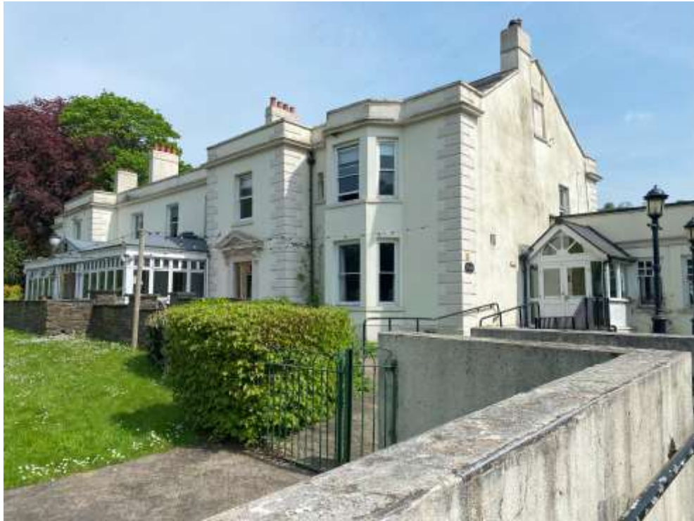
Plate 7 – West frontage of Pentrebach House with later conservatory addition to centre and single storey extension to the right of the image.
