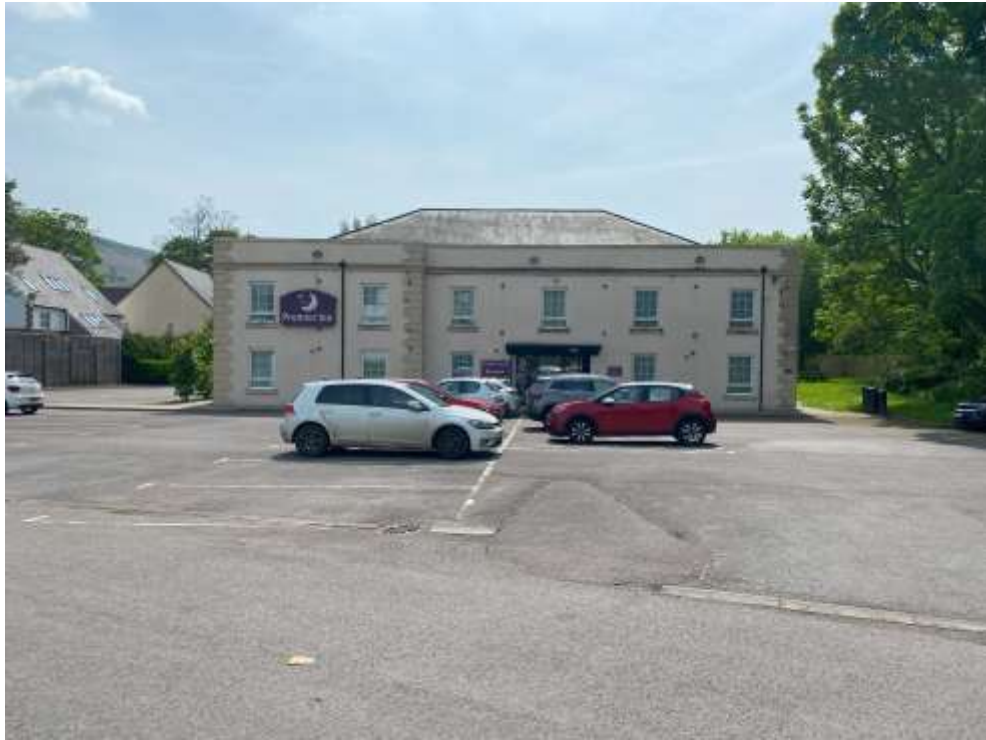
Plate 5 – North elevation of the extant hotel block; location of the proposed extension not visible.
