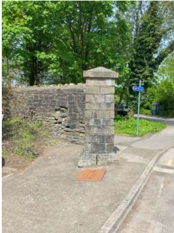
Plate 11 – Gate pier and boundary wall to the north of the Site.
