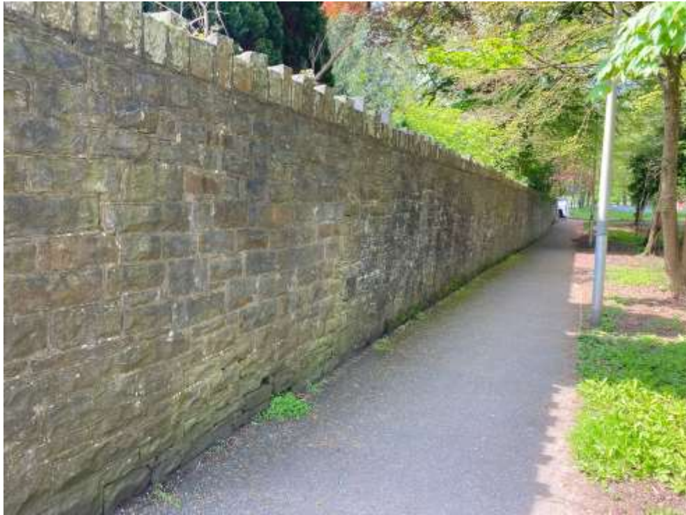
Plate 13 – North face of the Grade II listed boundary wall along the north and northwest of the Site frontage.
