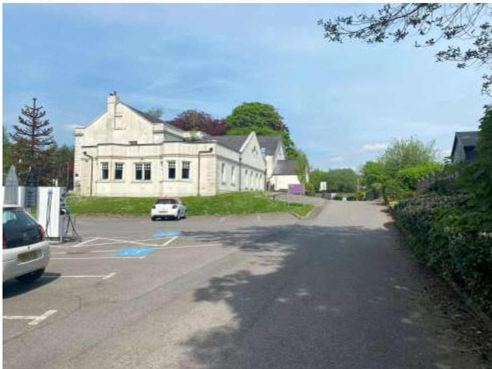
Plate 8 – South and part east elevations of Pentrebach House showing later additions and alterations.
