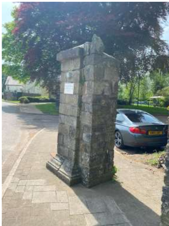
Plate 12 – North face of gate pier.
