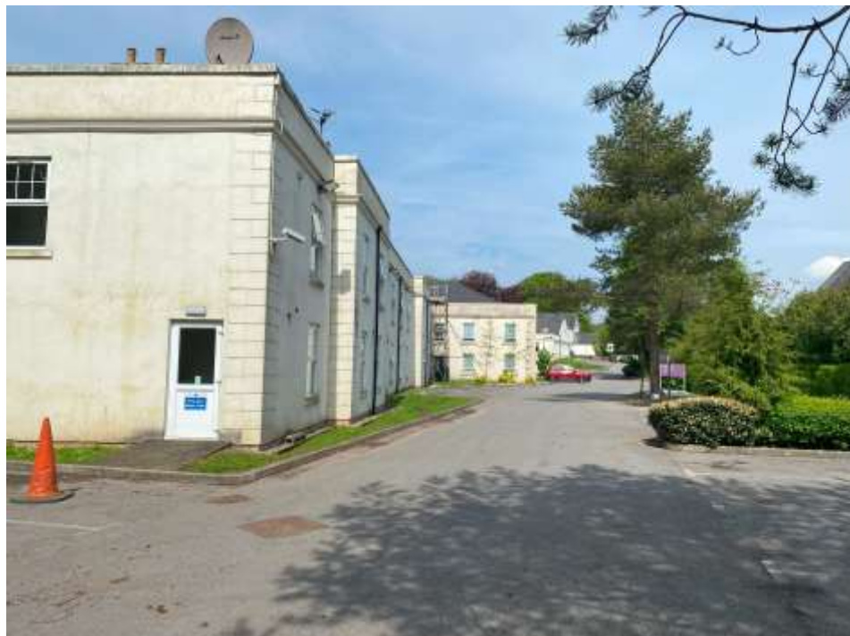
Plate 2 – East and part south elevations of the extant hotel block viewed on the site of the proposed extension.
