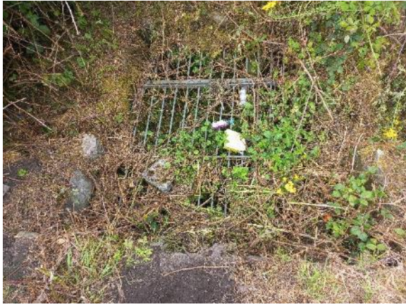
Culvert within dense bramble (see Target Note, Plan 2)
