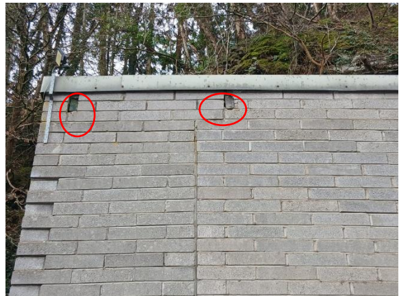
Photo 4: Cracks in the Rendering
