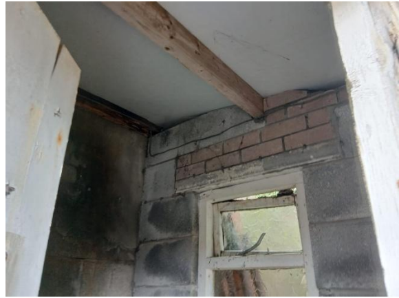
Photo 14: Gaps in the Rendered Wall
