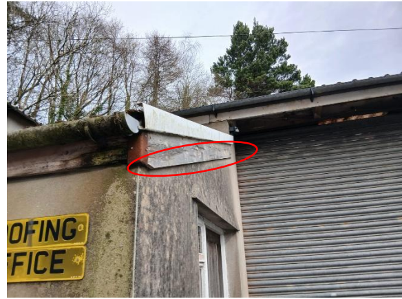
Photo 8: Raised Lead Flashing
