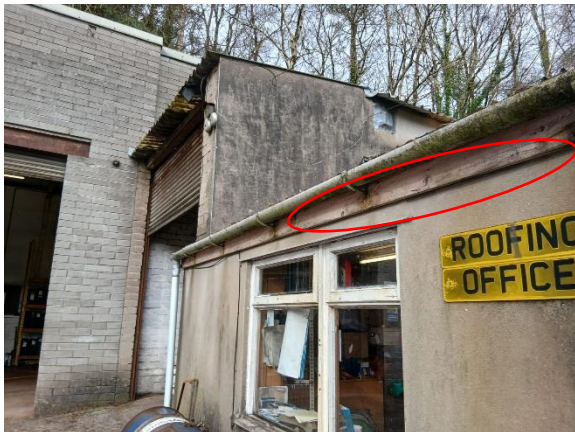
Photo 3: Raised Bargeboards in the Eastern Elevation
