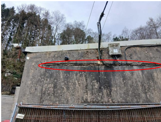
Photo 9: Cracks in the Rendered Walls
