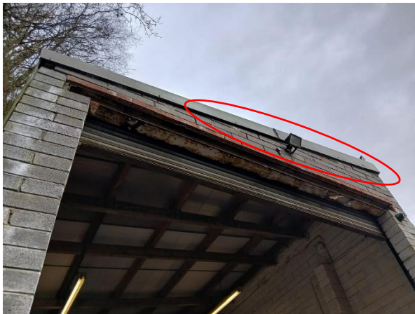
Photo 3: Raised Bargeboards in the Eastern Elevation
