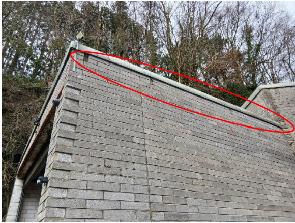
Photo 7: Gap in the Bargeboard
