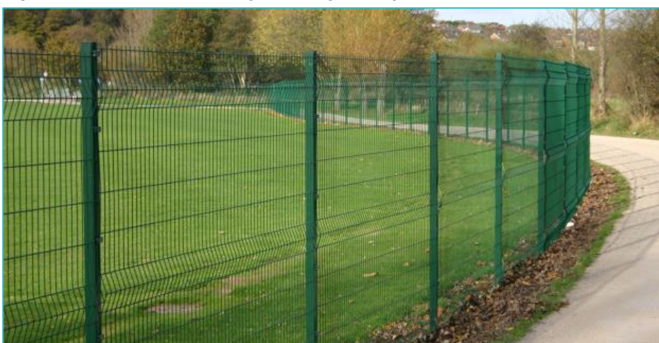
Figure 4: Weldmesh Security Fencing Example
