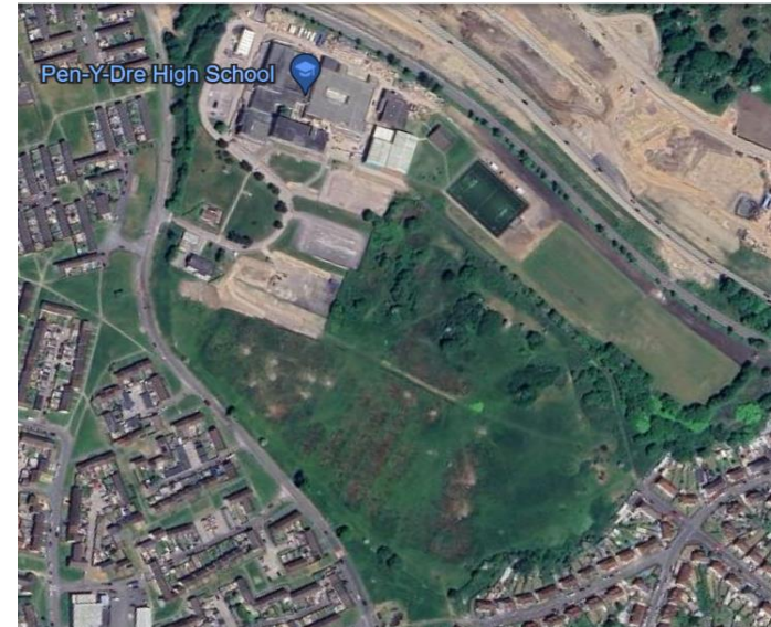
Fig.1.2 – Aerial View of the proposed School site including Pen Y Dre and the lower field where the new build will take place.
