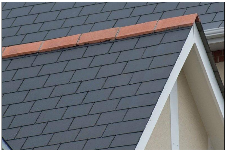
1 Marley Fibre Cement slate
