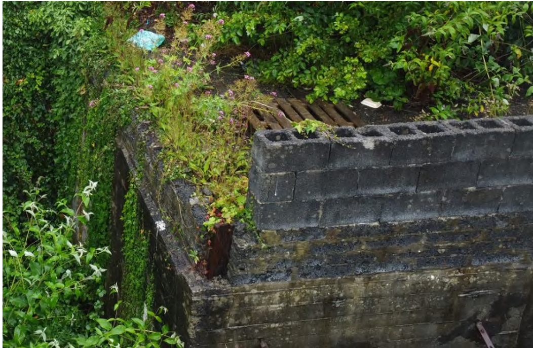
Plate 5 showing the site retaining walls
