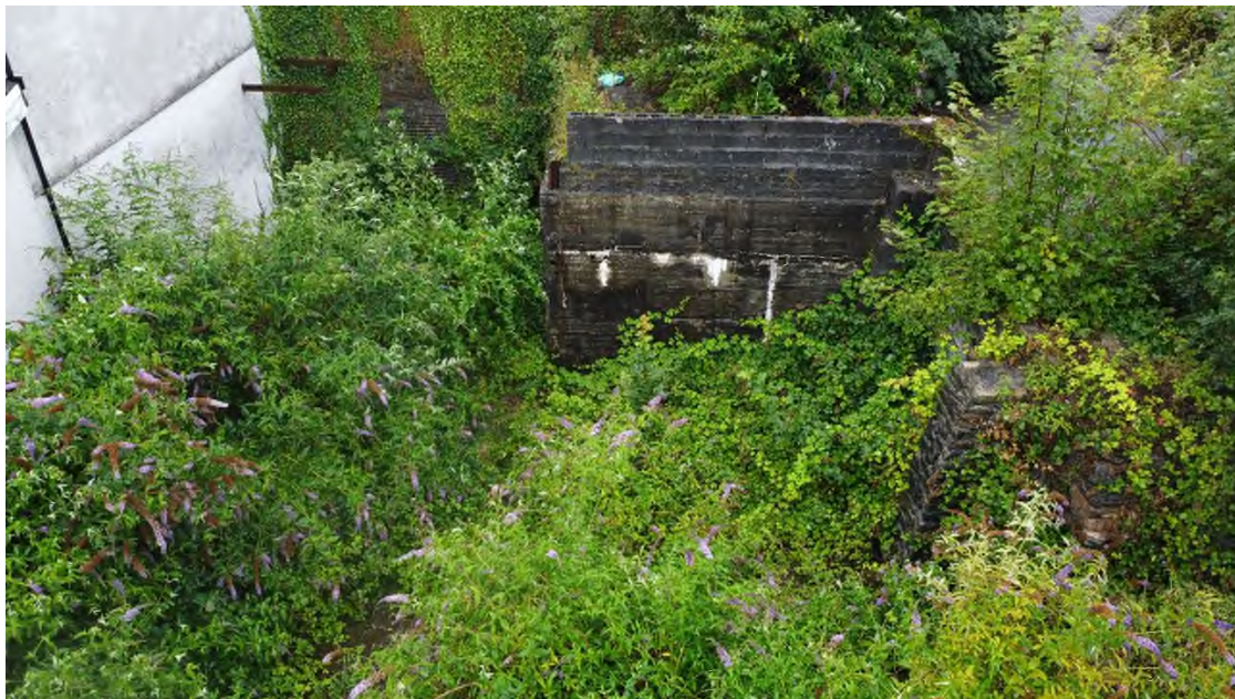
Plate 4 showing site interior with scrub dominating the site
