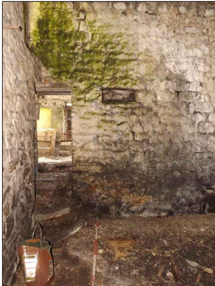
Plate 18. West elevation of the barn inside Annexe 1 showing the access doorway into the barn interior and the engineered recess in the wall. Note the line of stones at the top of the image indicating the line of the former roof of the barn prior to its level being raised. Scale 2m.
