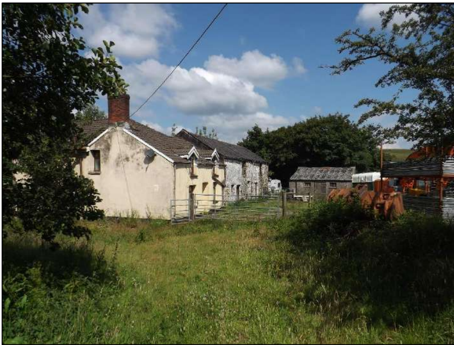
Plate 49. General view of Tynycoedcae Farm from the original access track.
