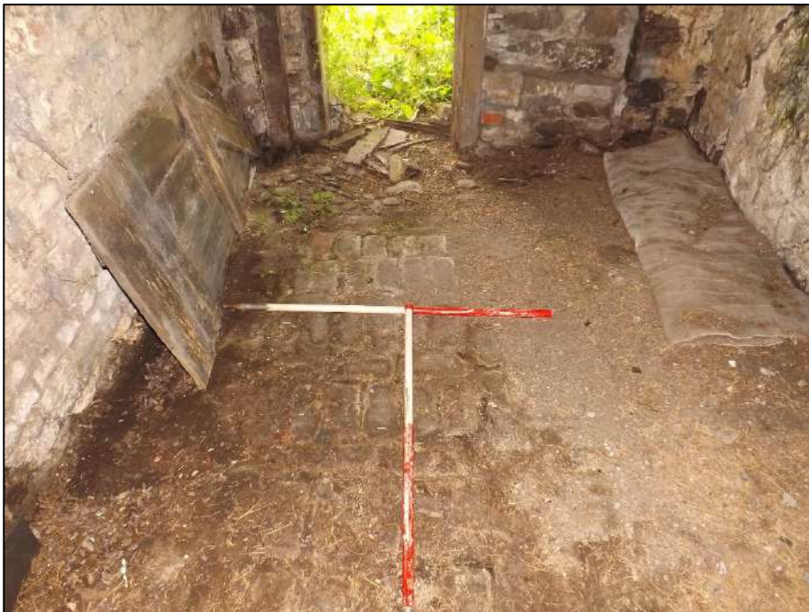
Plate 25. Brick and cobble floor of Annexe 3. Scale 1m.
