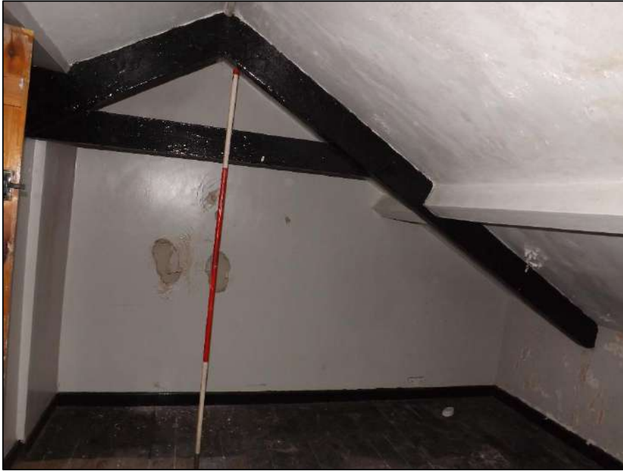
Plate 42. Heavily painted roof beams in the south east bedroom. The beams were tied with metal bolts but although hidden under layers of paint, they are likely to be original beams dating to creation of the cottage. Scale 2m.
