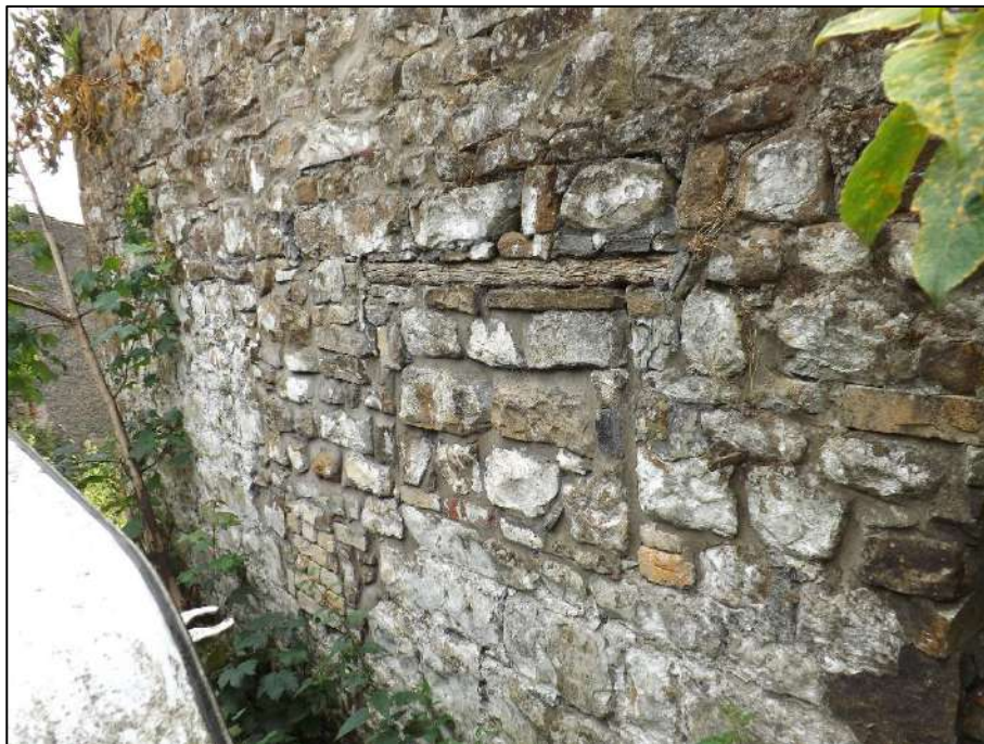
Plate 14. General oblique view of blocking of a window at the lower level of the north elevation of the barn. Note the timber lintel.
