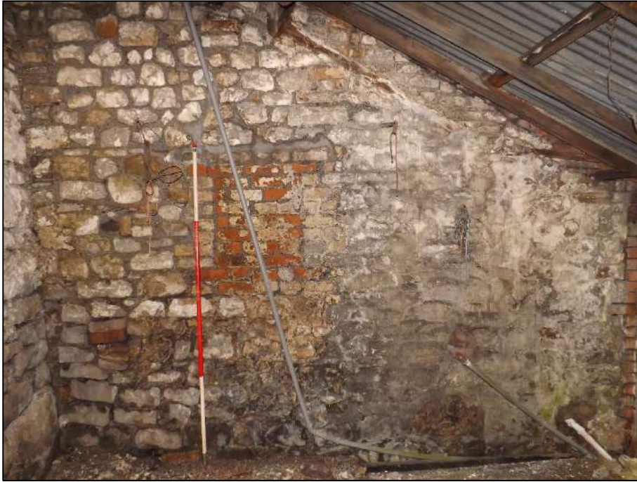
Plate 17. South wall of Annexe 1 showing possible blocked window and old roof line. This wall, which forms part of the north wall of the cottage, was not keyed into the barn wall. Scale 2m.
