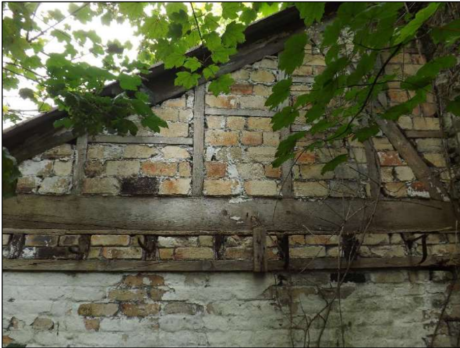
Plate 20. North wall of Annexe 2 showing timber frame and brick infill construction of the upper part of the wall. Note the metal fixings which may have been for hanging implements.
