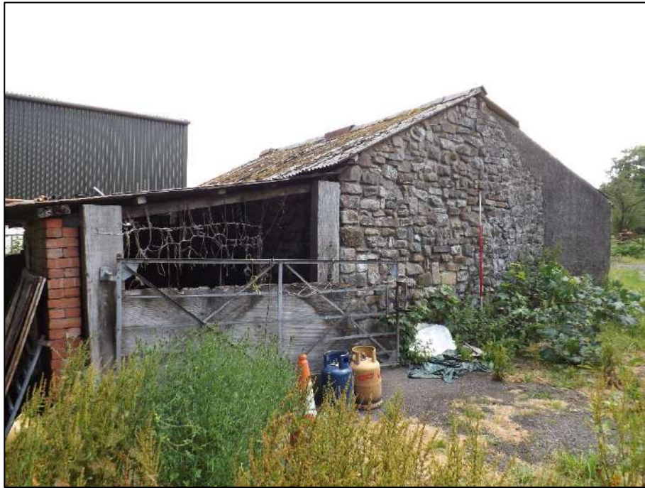
Plate 2. West elevation oblique view showing first phase construction (stone) second phase (pebble dash render) and open sided extension to the north. Scale 2m.
