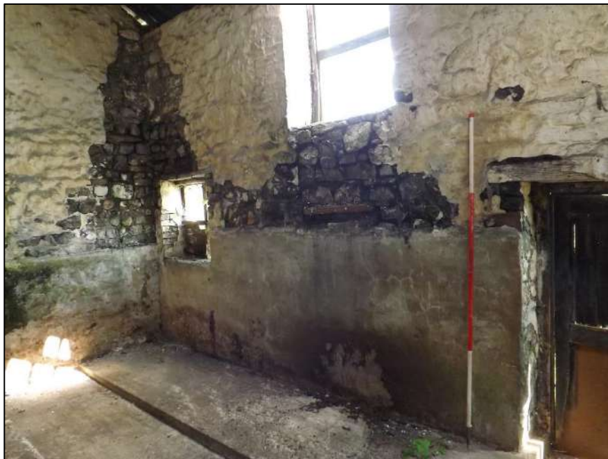
Plate 29. Oblique view of the north east interior of the barn. Note the original sill for the partially blocked upper window and the former doorway in the corner that had been converted into a window. Scale 2m.
