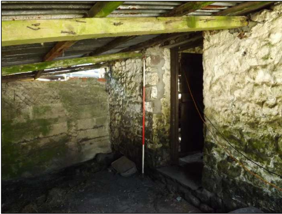
Plate 4. Oblique view of the original first phase north elevation, now contained within a later extension. Note reinforced concrete render to reverse of the old boundary wall. Scale 2m.
