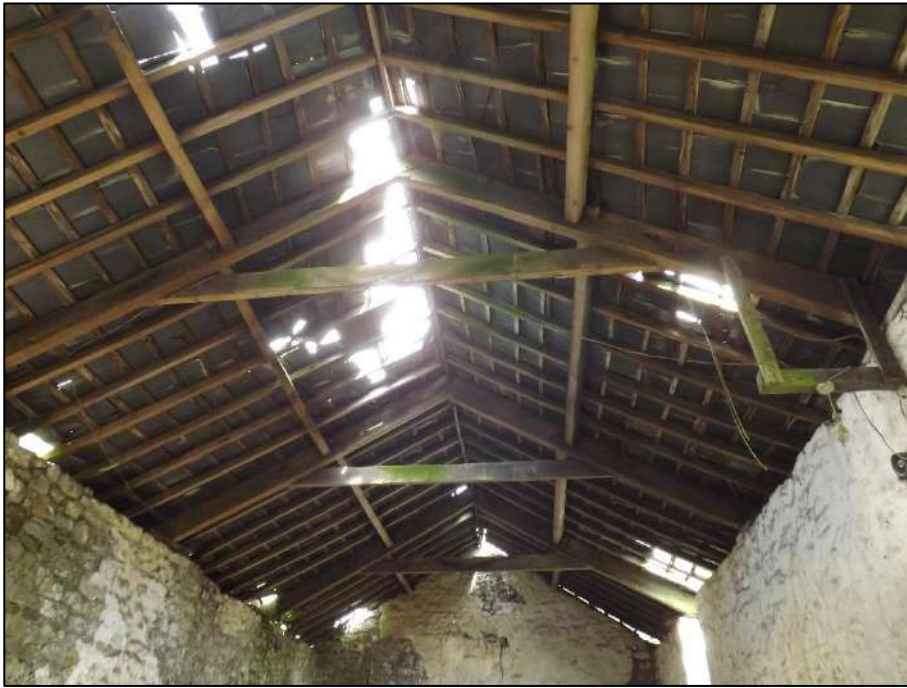
Plate 30. Detail of the roof construction of the barn interior. Note the slates have been affixed directly onto the timber. It is unclear as to whether this is the original roof but it is certainly of some age and may date to the re-modelling of the farm before 1875.
