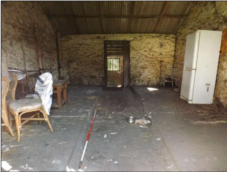
Plate 7. Interior view of the hen house towards the north, looking towards the original doorway. Note the raised floor levels. Scale 2m.
