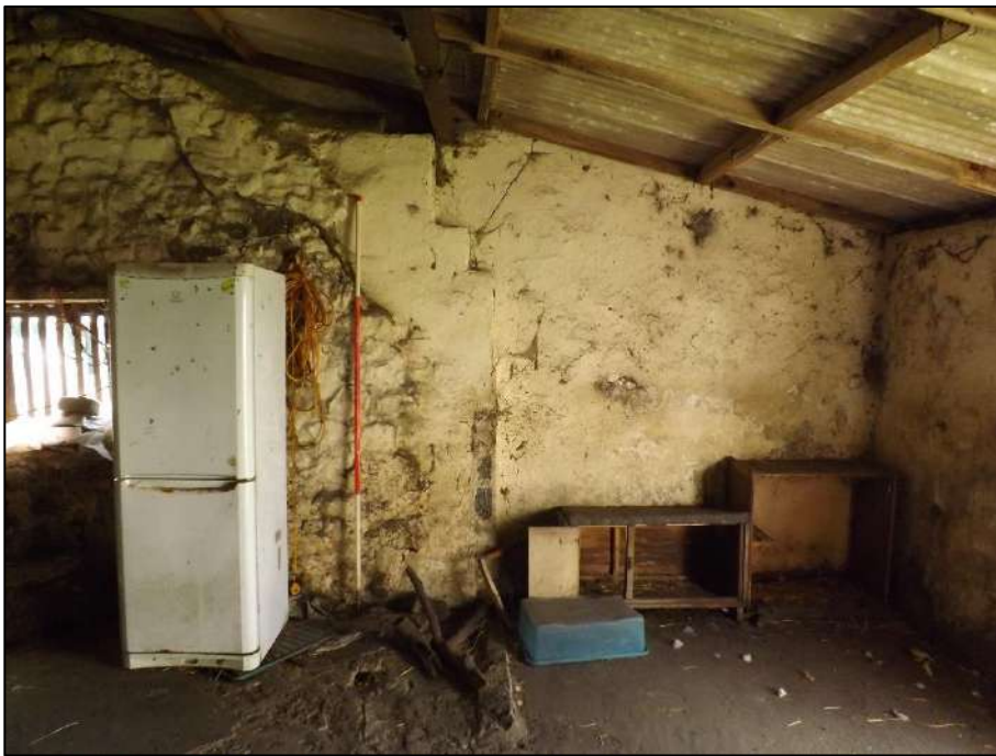
Plate 8. Internal view of the east elevation showing the construction of the second phase extension. Note the remains of a breeze block partition to the left of the blue box. Scale 2m
