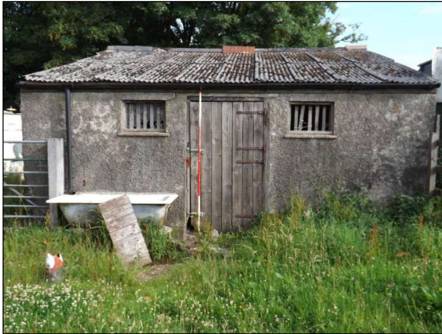
Plate 1. South elevation of the hen house. Scale 2m.
