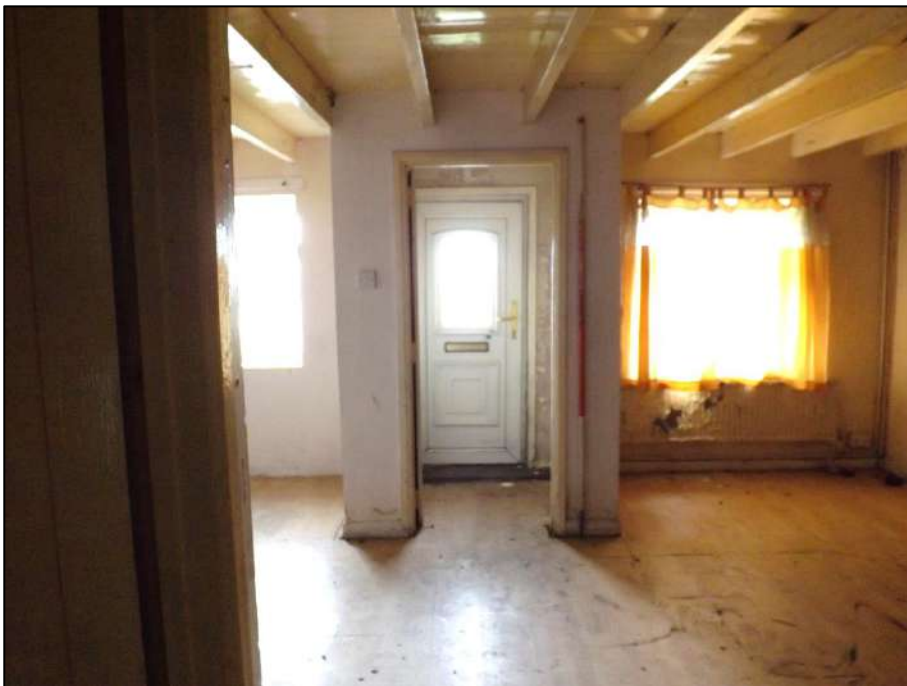
Plate 38. Internal porch and exposed ceiling beams in the living room. Scale 2m.
