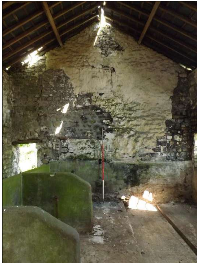
Plate 28. North wall of the barn interior. Note the blocked window in the upper level of the gable and the concrete render that extended round from the byre. Scale 1m.
