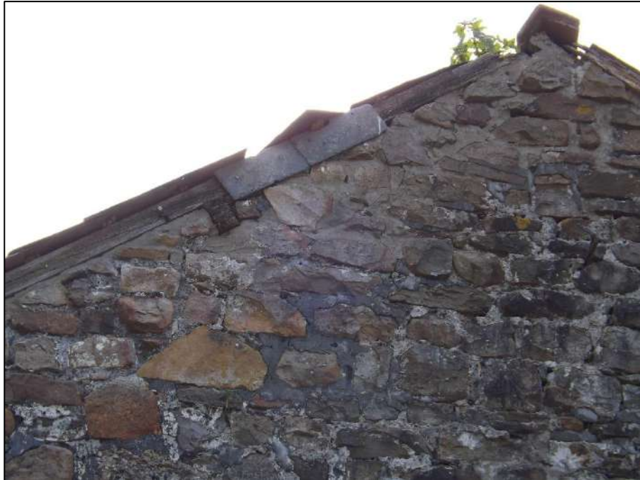
Plate 15. The former roofline was visible in the north gable of the barn. Note the remains of two slates nailed to the end roof joist as a weather board.
