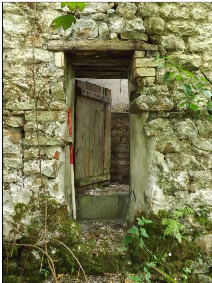
Plate 21. Interior door from Annexe 2 to the barn showing the step and doorway. Scale 1m.
