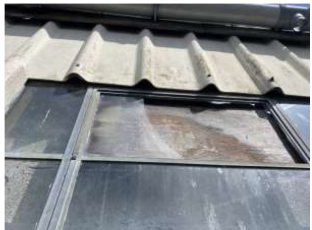
Photo 10: Southern Elevation Window Gaps
