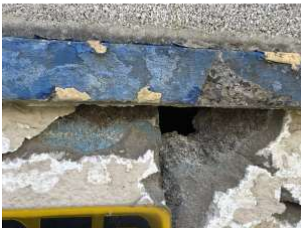
Photo 9: Cavity in External Wall Northern Front
