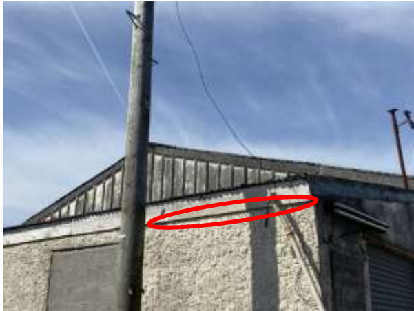
Photo 9: Cavity in External Wall Northern Front
