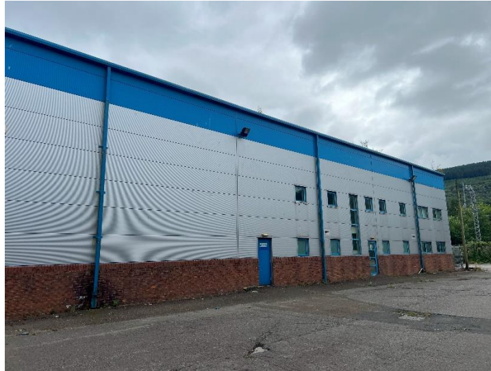
Photo 9: overview of the external structure of building 2
