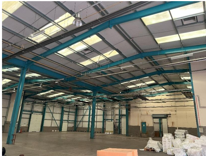
Photo 10: Overview of the internal structure of building 2.
