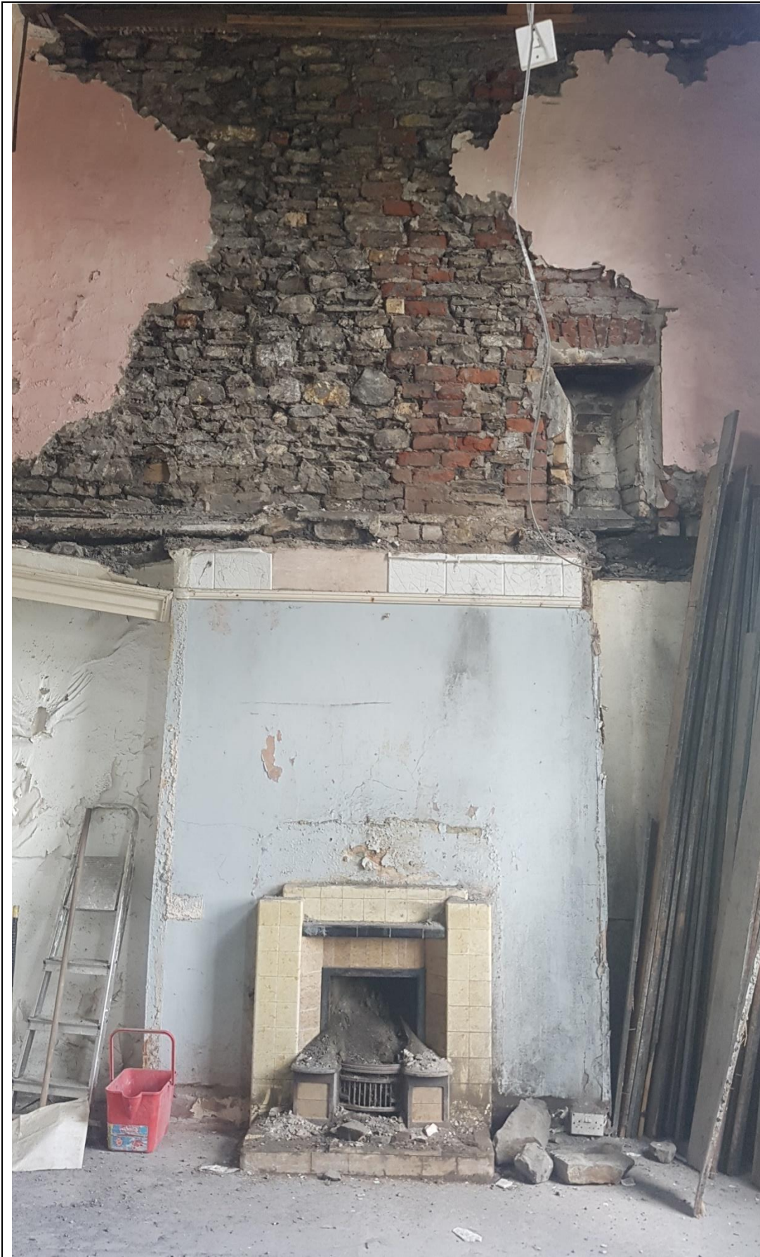
Photo 7. Ground and former first floor interior
