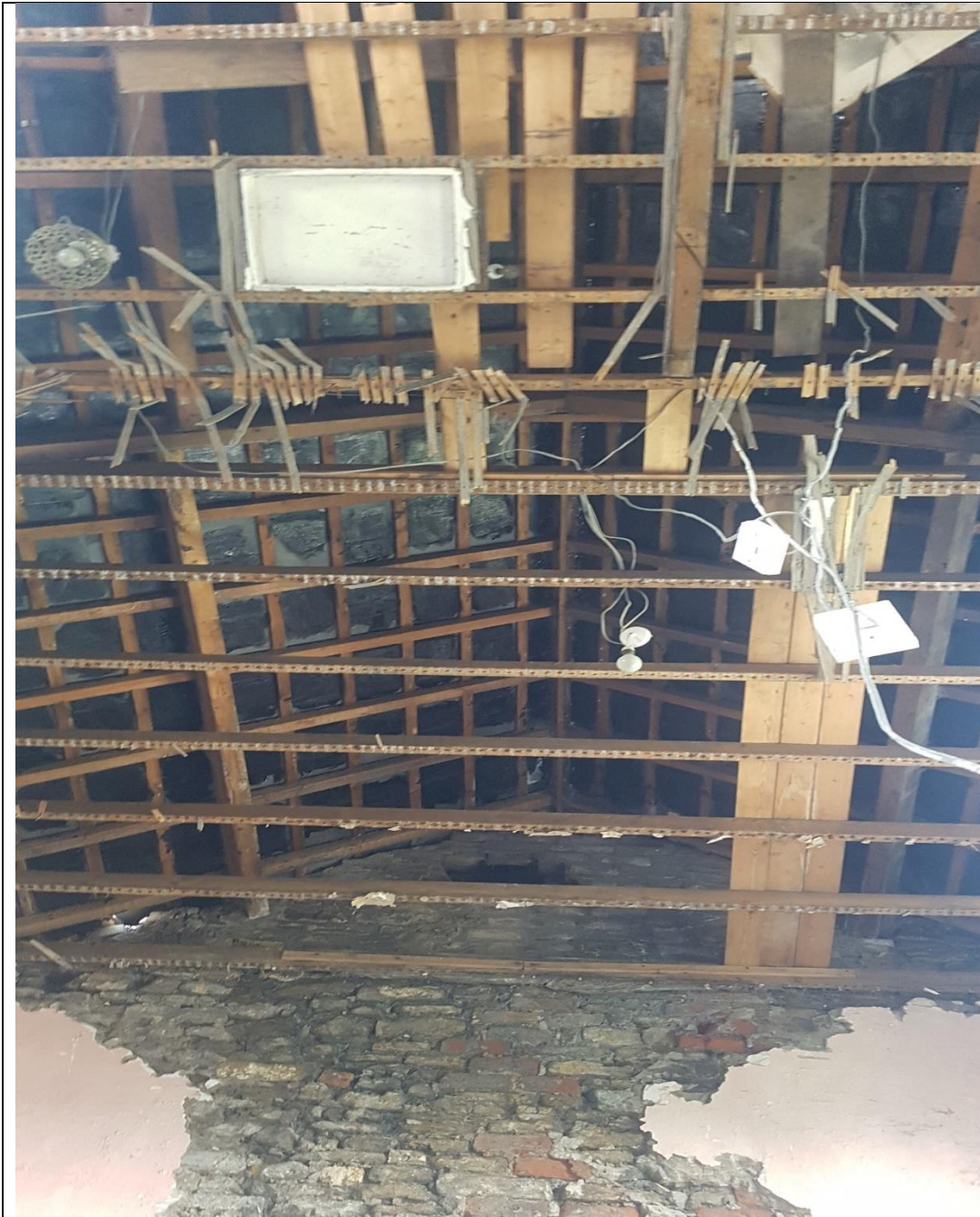
Photo 6. Underside of the roof covering
