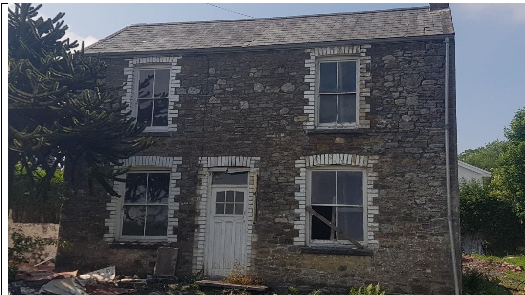
Photo 1. Front elevation of Waunfach House (north). Windowpane opened on survey day by owners, but usually covered by board. Covered on both dusk visits.
