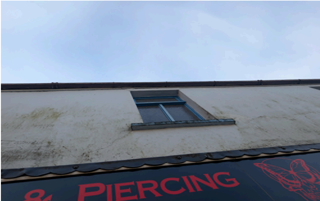
Plate 3 – Photograph of front elevation fascias
