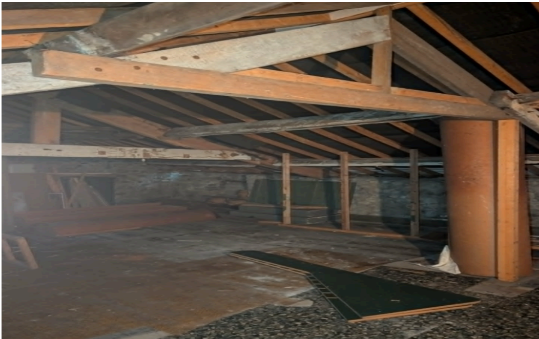
Plate 1 – Photograph of roof void
