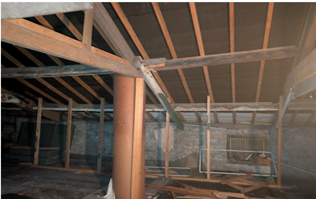
Plate 2 – Photograph of roof void
