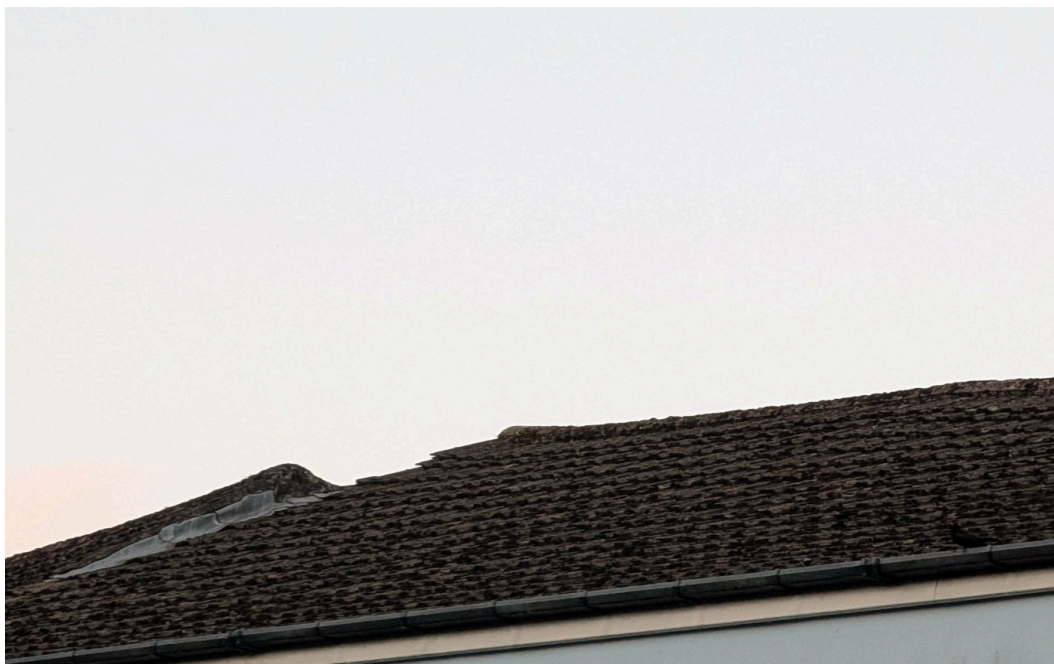
Plate 7 – Example of tight fitting tiles
