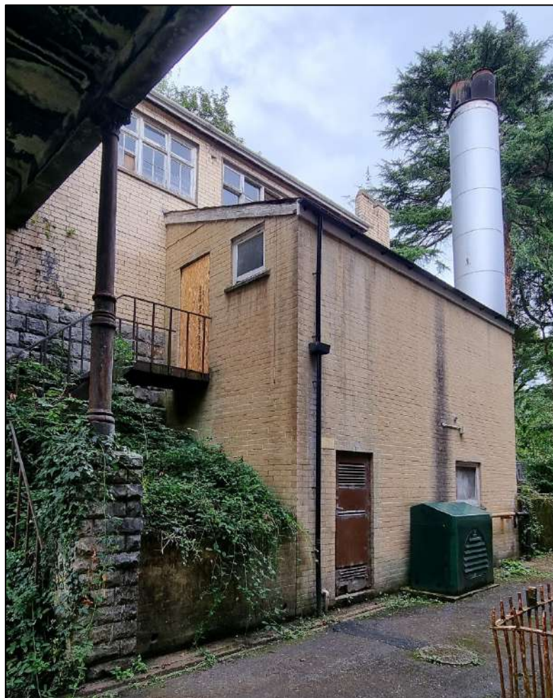
Plate 7: Boiler Room to basement level of lean-to section, looking east.
