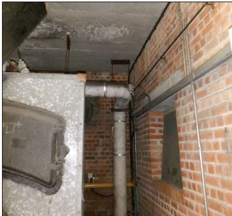
Plate 11. Blocked window with cement lintel on south-west wall to righthand side, looking south-east.
