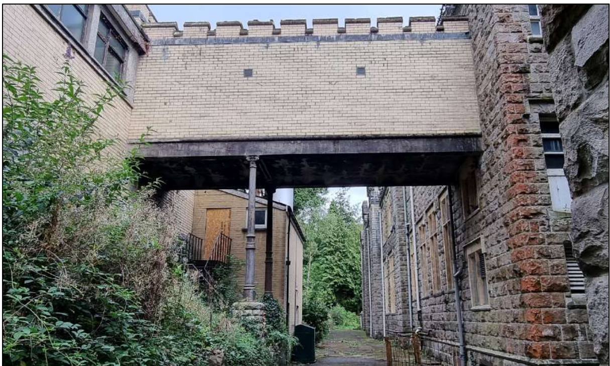
Plate 5. Covered walkway between rear of Cyfarthfa Castle rear building, looking south-east.
