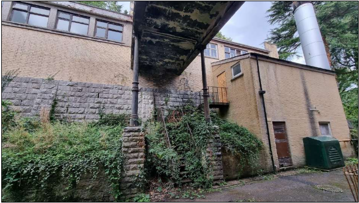
Plate 6. Attached building to the rear of the Castle, including Boiler Room to the righthand side. Looking north-east.
