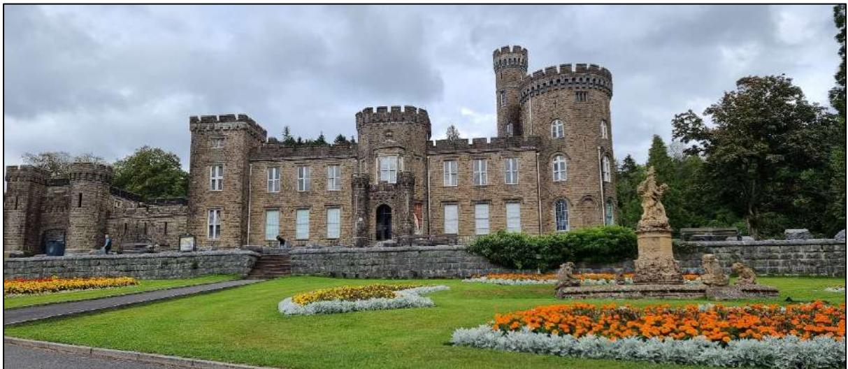
Plate 2. Front (south-west) facing elevation of Cyfarthfa Castle, looking north-east.
