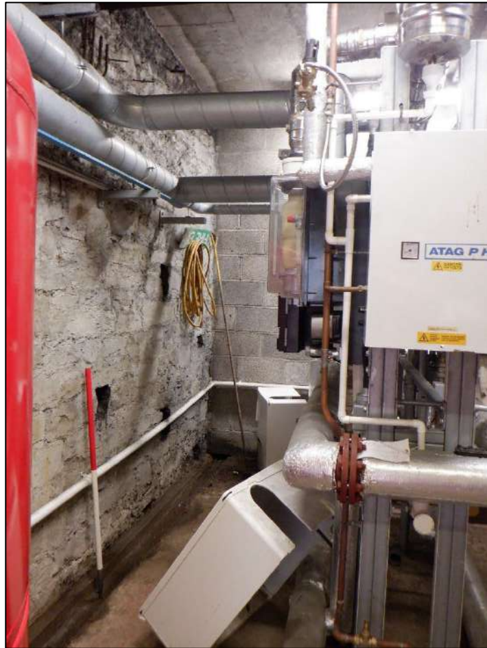
Plate 10. Rubble stone north-west wall and aerated block north-east wall, looking north-east. 1m scale.
