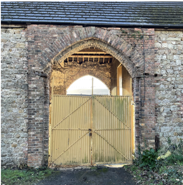
Photograph of existing archway
