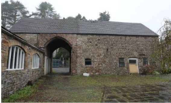
Fig.75 South elevation. Offset tall carriageway with pointed arch in brick contrasts with the coursed rubblestone – perhaps this has been inserted? Domestic scale openings at ground floor level with brick arched heads and later 20 th century windows and door.
