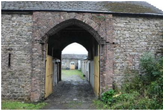
Fig.78 The carriageway with well worn stone sett floor. The corrugated iron doors are modest compared to the huge doors that must have once graced the openings on both sides denoted by the heavyweight iron sockets for the original doors.
