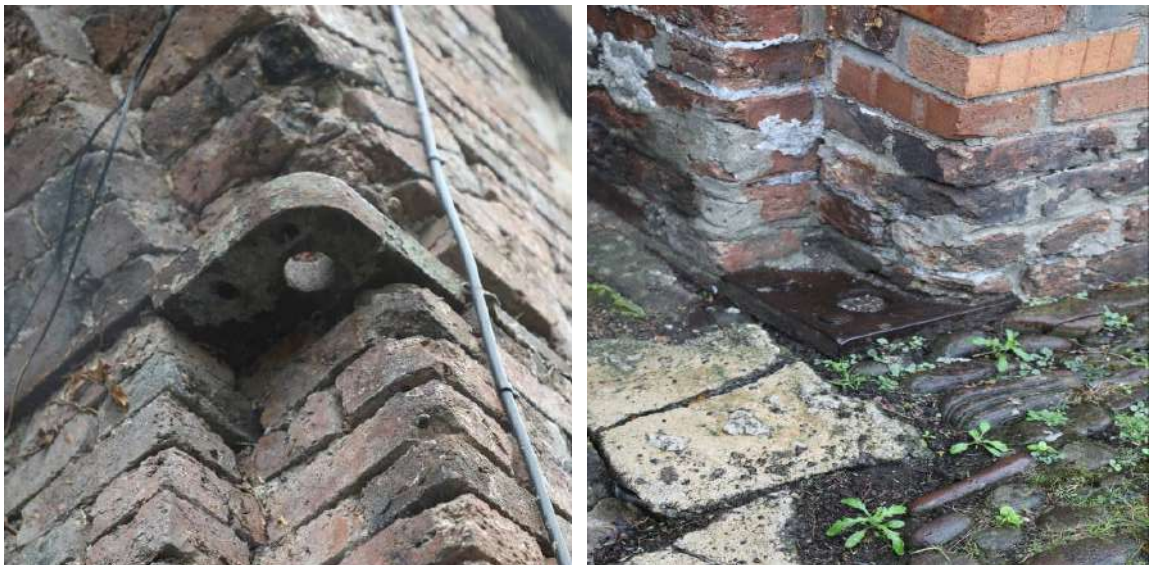
Fig.79 The heavyweight iron sockets for the original opening doors found on both sides of the carriageway.
