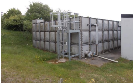
Plate 3: the water tank adjacent to the site. This structure has been judged to have negligible potential to support roosting bats. It will remain undamaged and in situ during the project. Photograph taken from the north-west.
