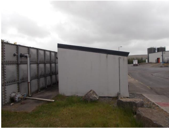
Plate 2: the small portacabin-like building adjacent to the site. This building has been judged to have negligible potential to support roosting bats. It will remain undamaged and in situ during the project. Photograph taken from the north.
