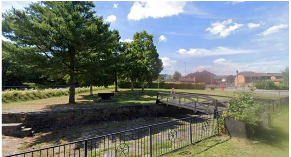
6 GM486 - Iron Canal Bridge from Rhydycar - View towards Pandy Farm
