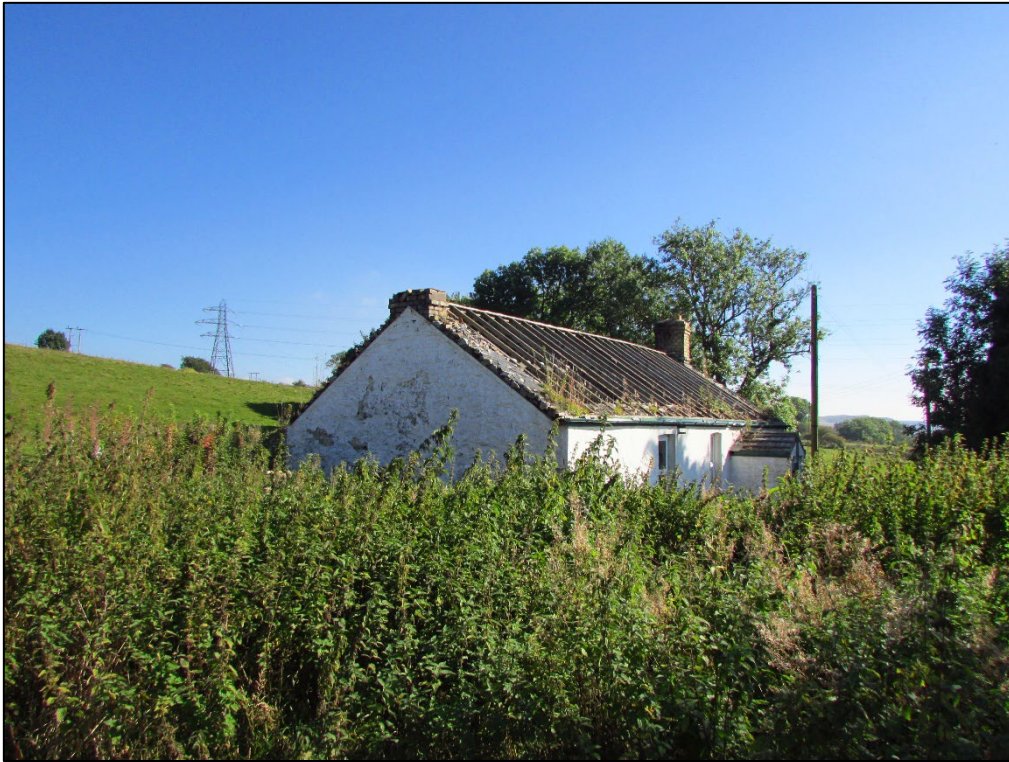
Photo 3: Grade II Listed Farmhouse in 2015 (north-west elevation)
