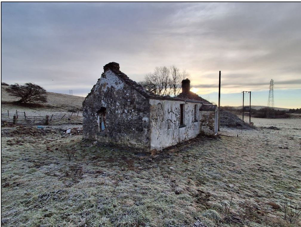
Photo 4: Grade II Listed Farmhouse in 2026 (north-west elevation)
