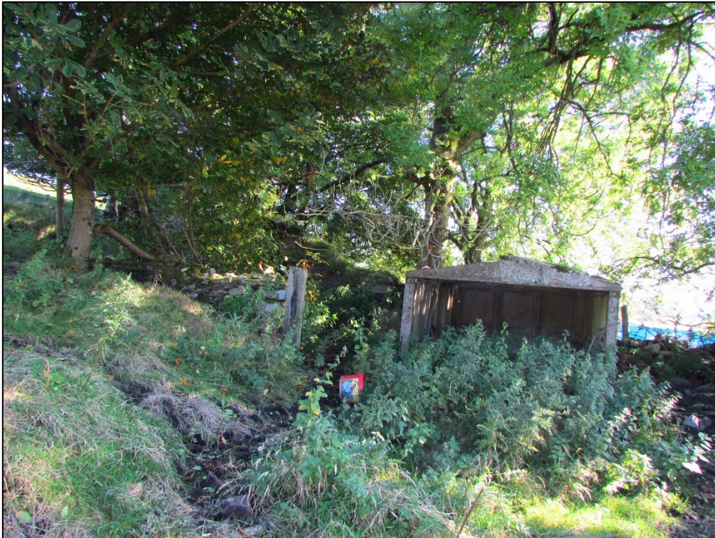
Photo 7: Barn to the south in 2015 (north elevation)
