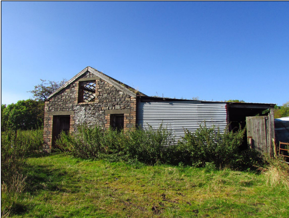
Photo 5: Barn to the north in 2015 (south elevation)
