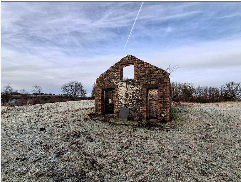
Photo 6 Barn to the north in 2026 (south elevation)
