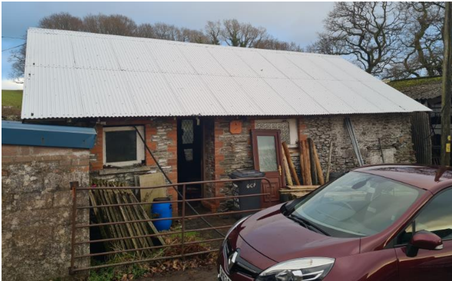
Photograph of Existing Building
