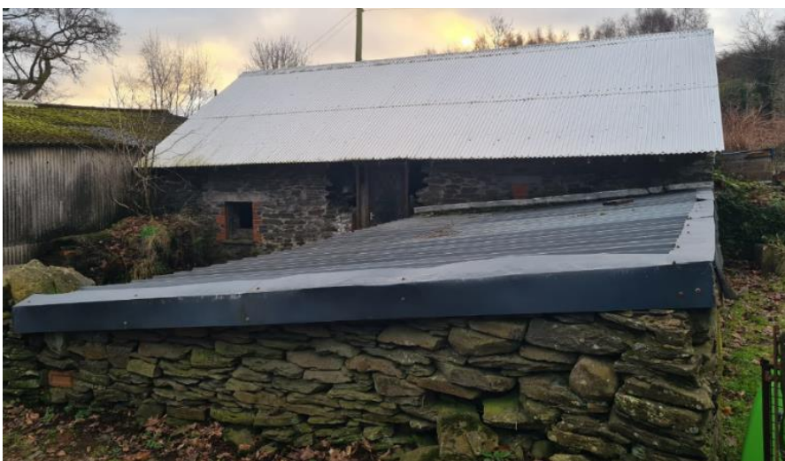
Photograph of Building from the Rear
