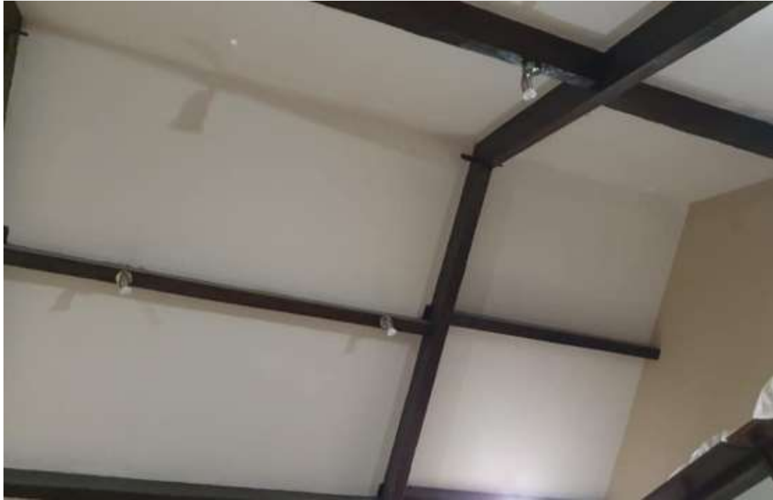
Plate 10- Photograph of vaulted ceiling
