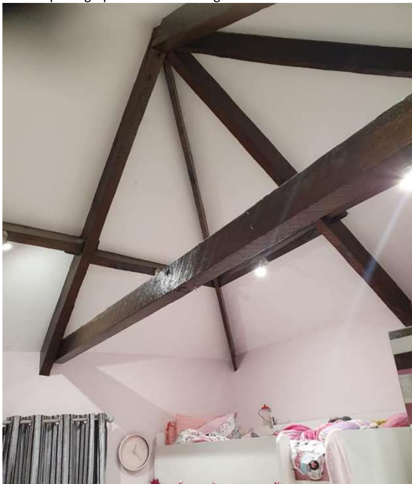
Plate 9- photograph of vaulted ceiling
