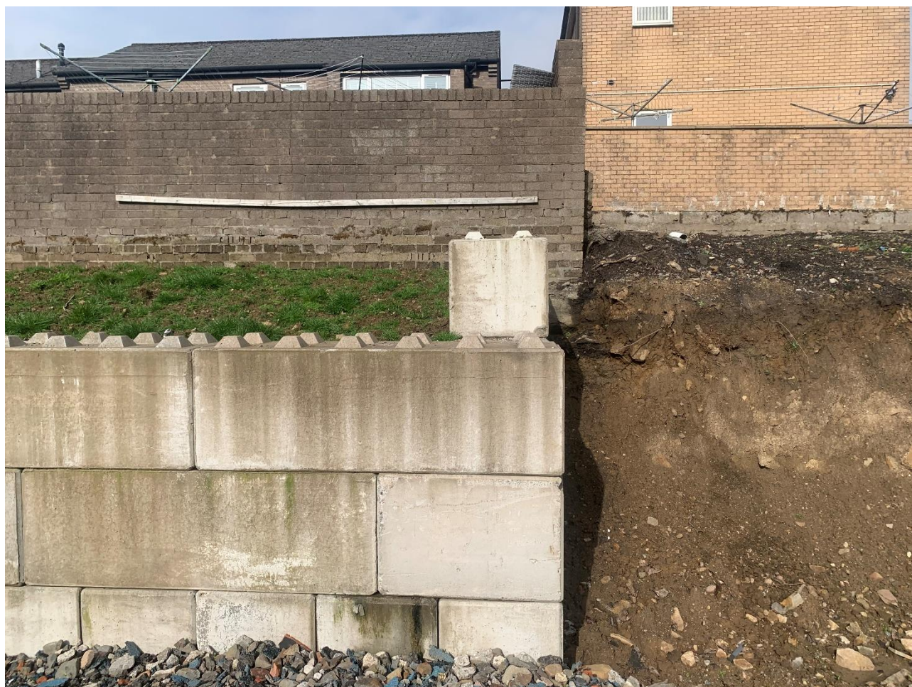
Photograph P11 - Wall Elevation 05-03-26
