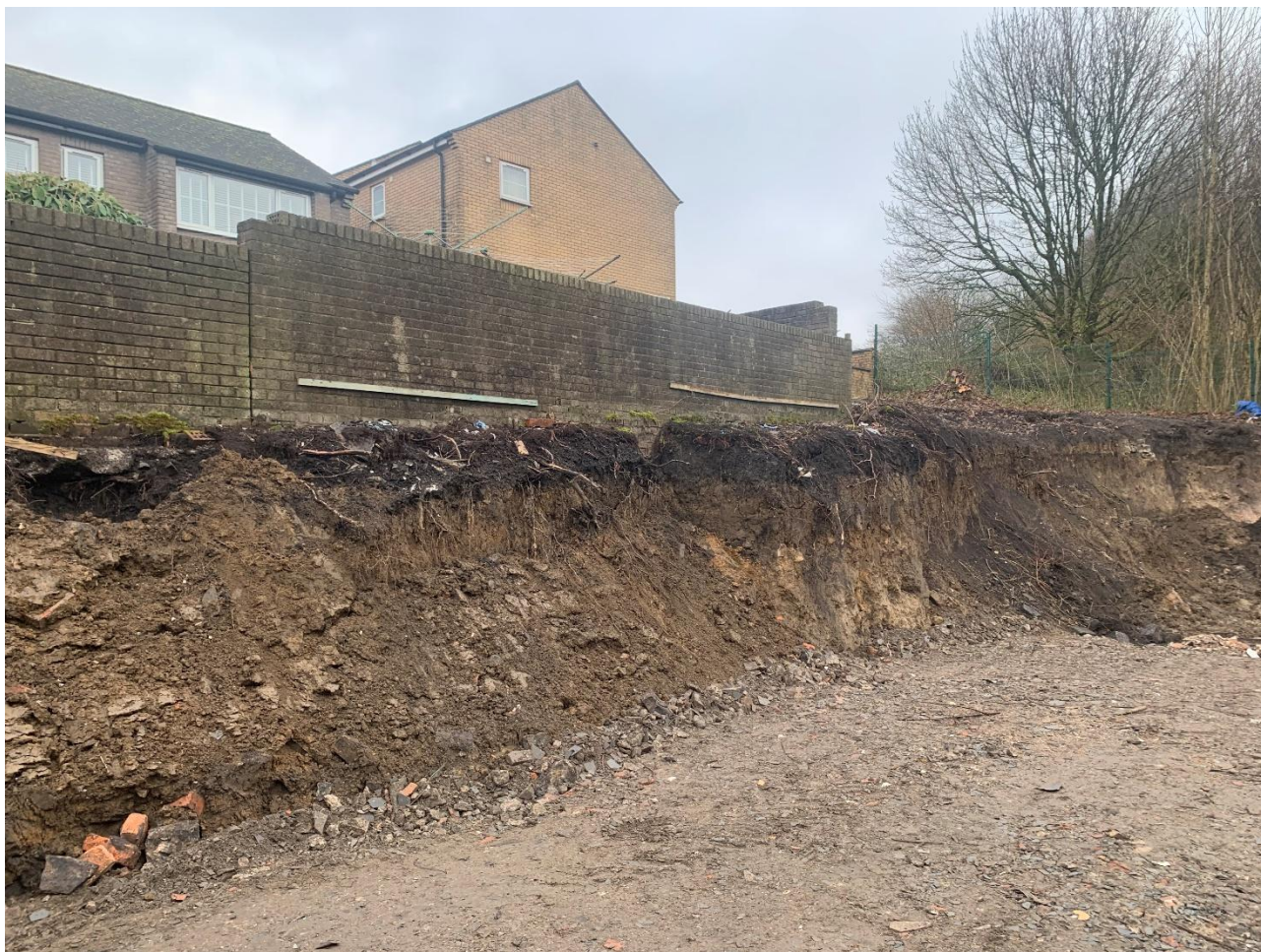
Photograph P5 – Wall Elevation 21-01-25
