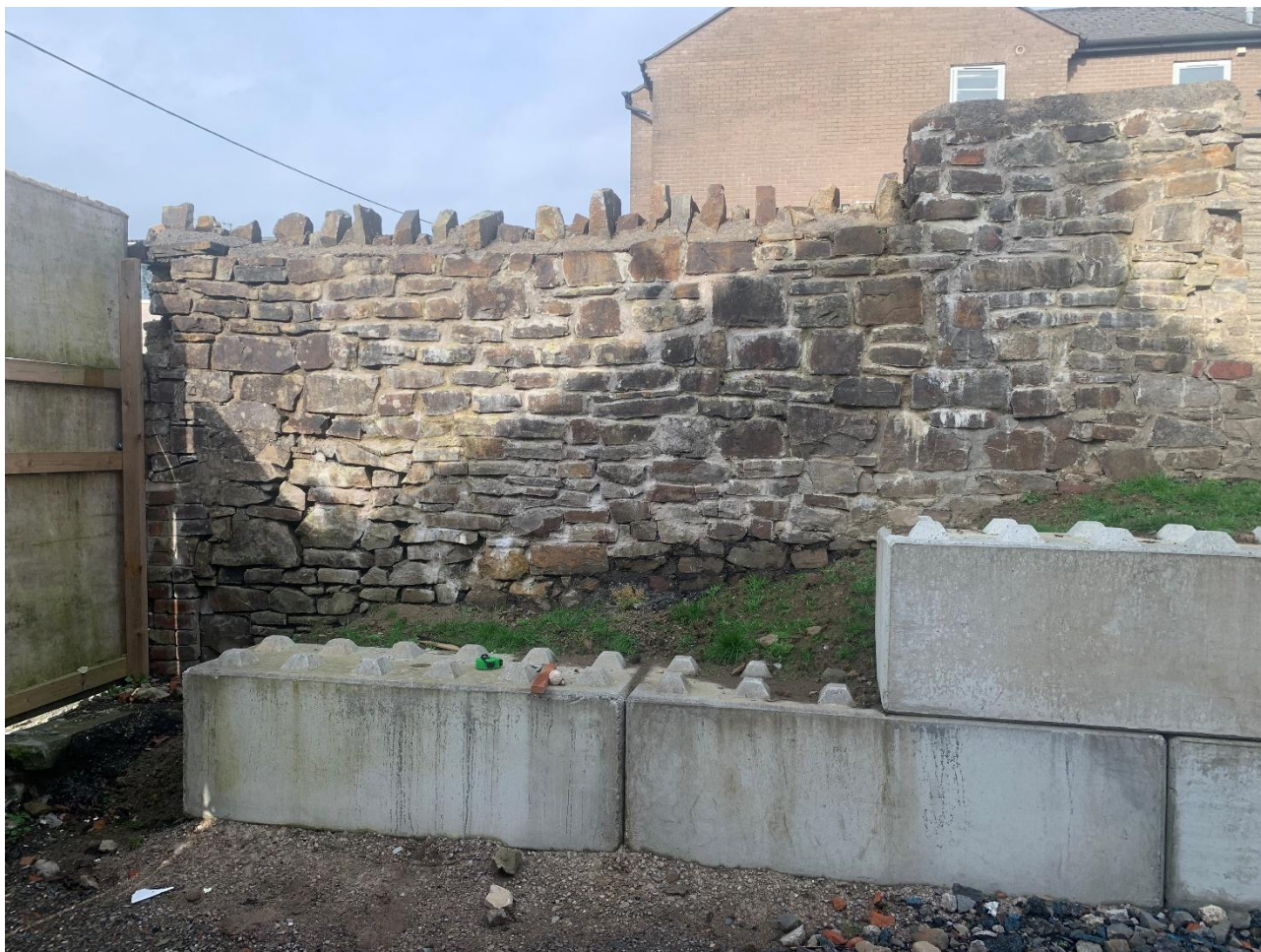
Photograph P7 - Wall Elevation 05-03-26
