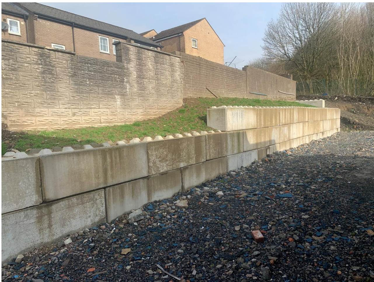
Photograph P9 - Wall Elevation 05-03-26
