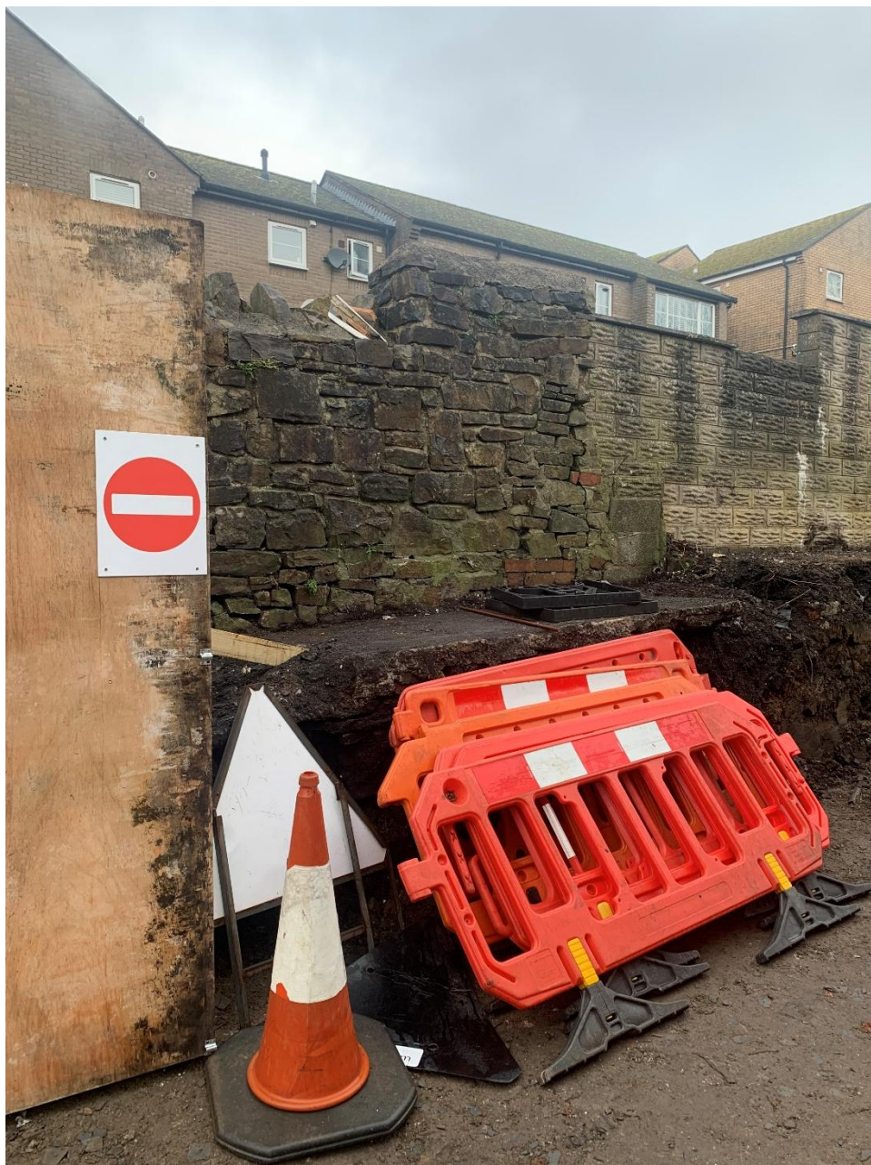
Photograph P1 – Wall Elevation 21-01-25
