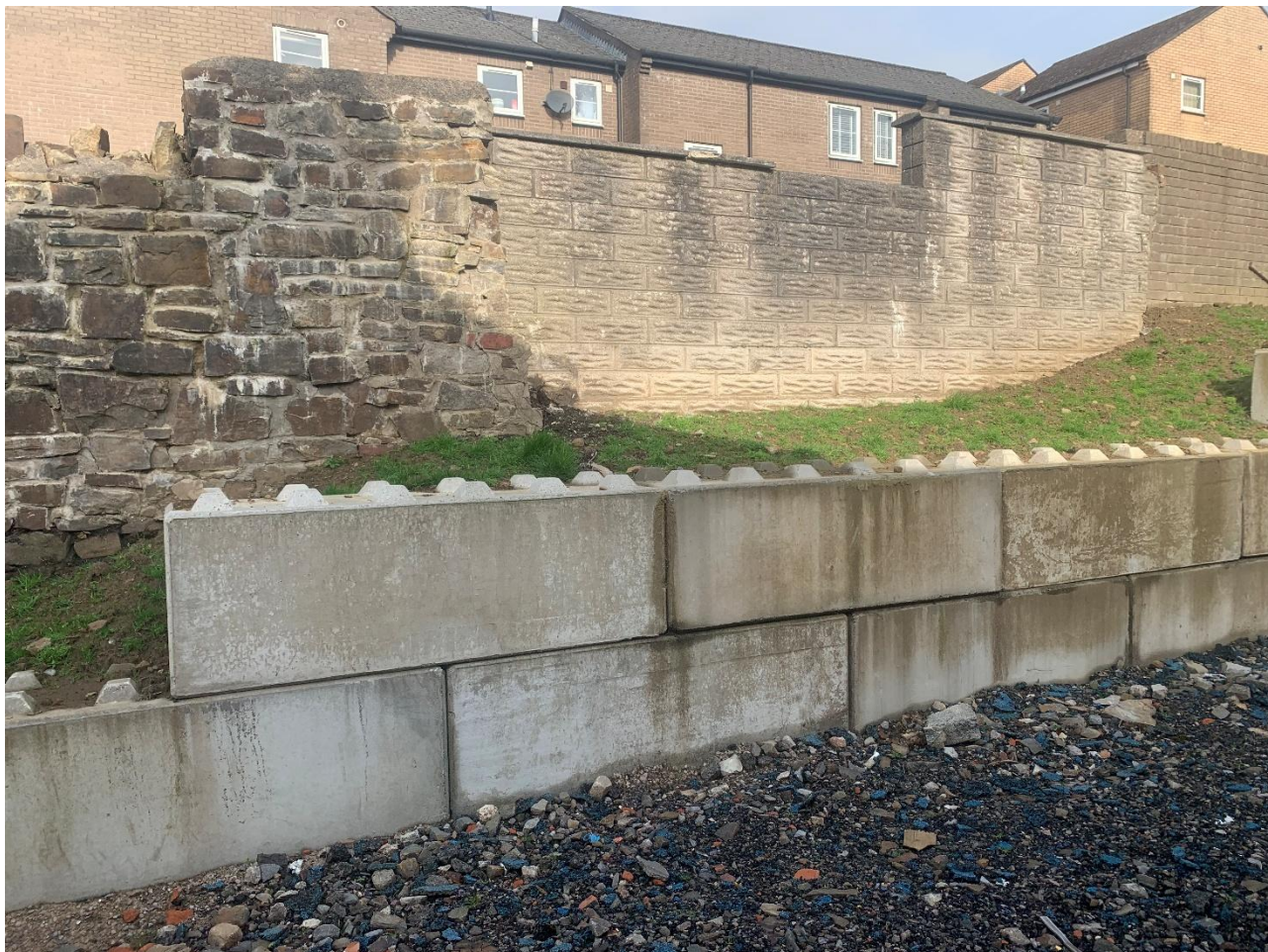
Photograph P 8 - Wall Elevation 05-03-26
