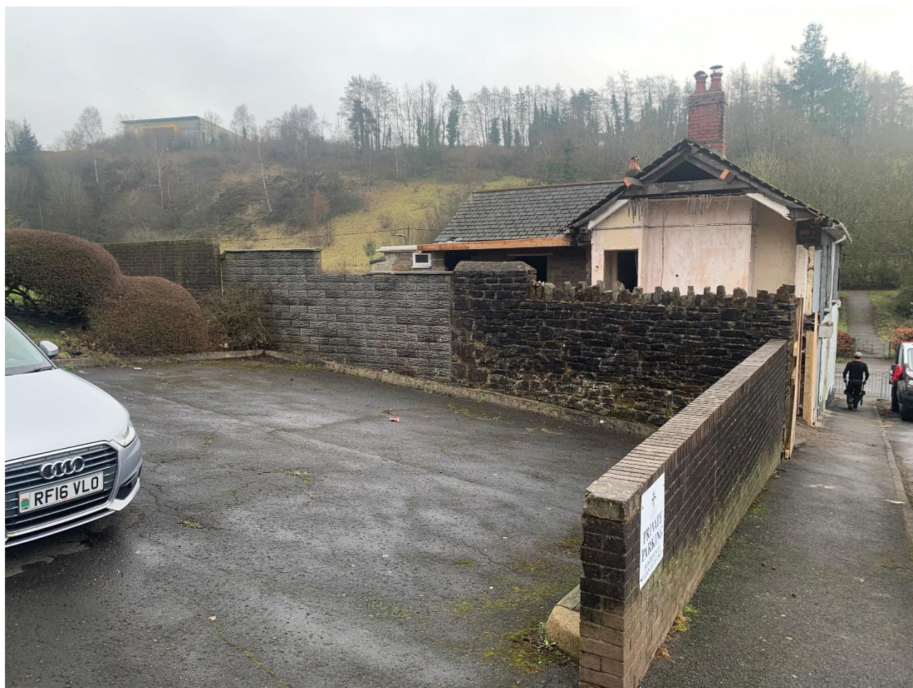
Photograph P6 - Neighbouring Land to the rear of Retaining Wall
