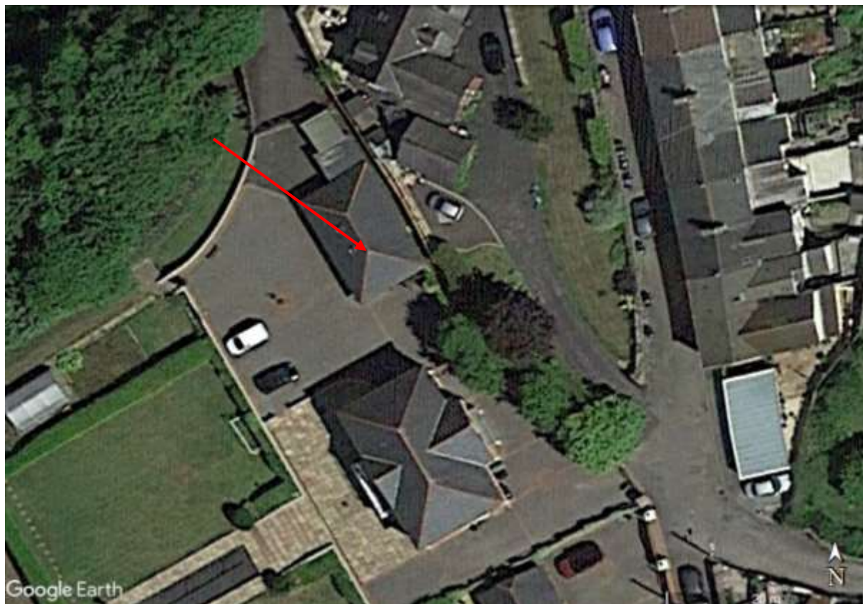
Figure 1: Detailed view of the garage (arrowed red)
