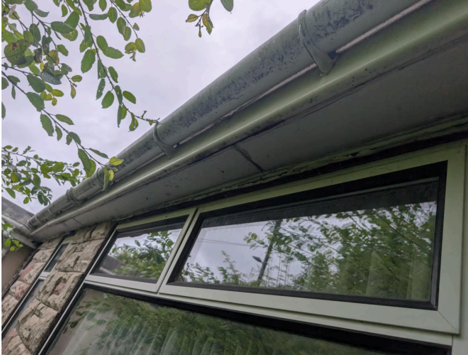
Plate 3- sealed eaves along rear elevation
