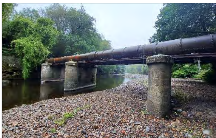
Photograph 5: River Taff flowing south -west under piers and iron feeder pipes left in situ following removal of the main bridge.
