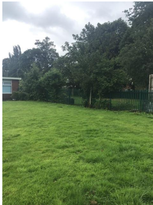
Image 9: Trees growing within fence line need to be removed before damage occurs.
