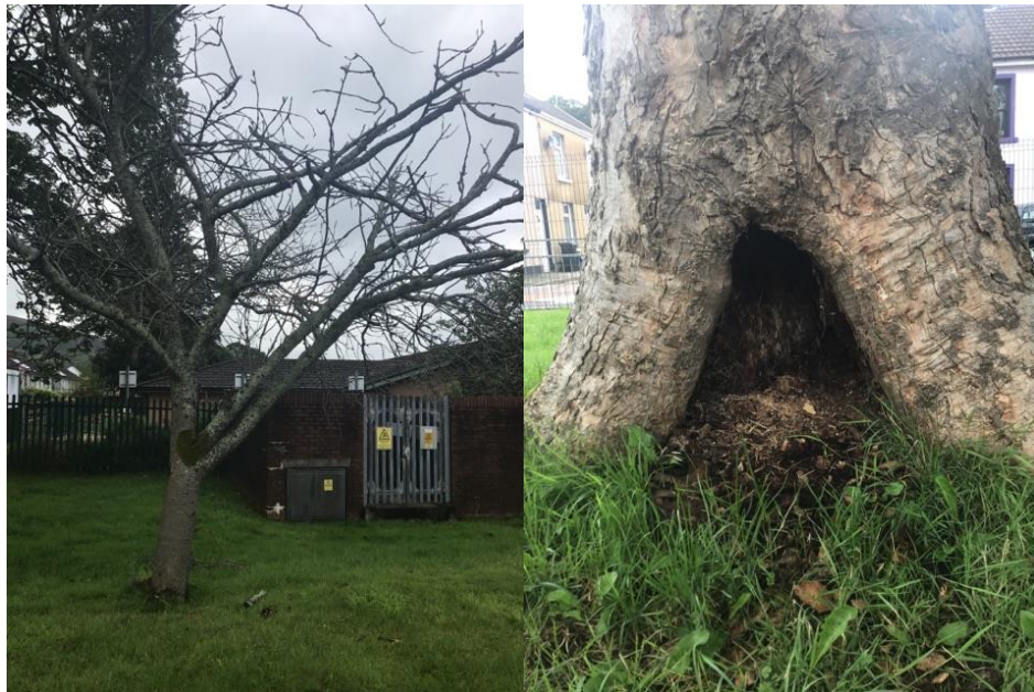
Image 1 and 2: Tree ID- 2463 and 2464: Hazardous trees for removal
