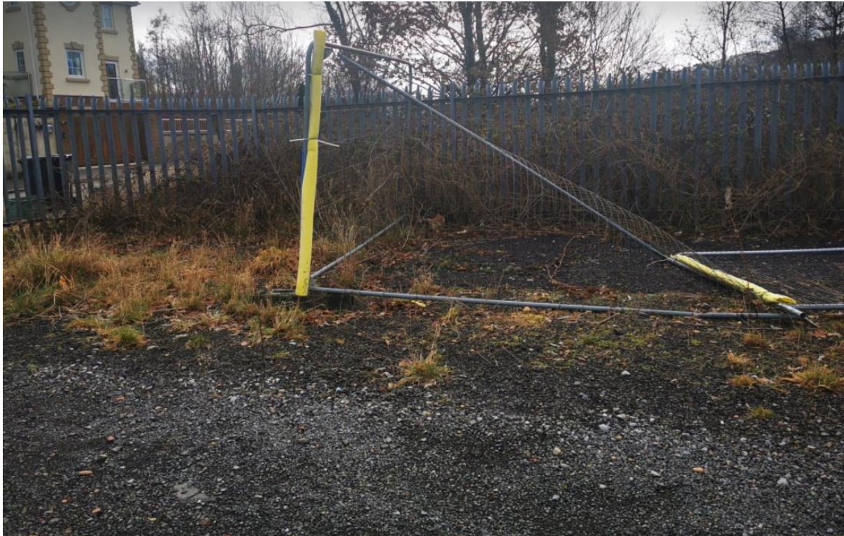
Plate 3- south eastern corner of the site
