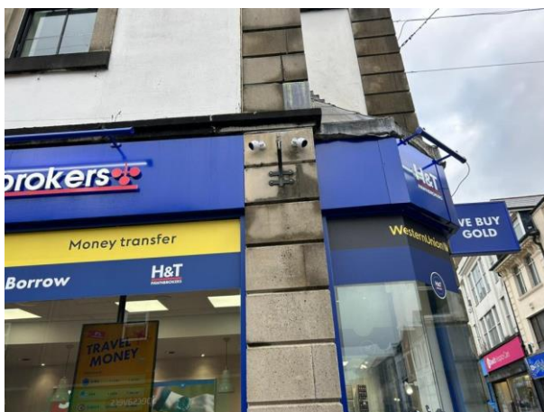
Photo 16: Shop Lighting Southern Elevation
