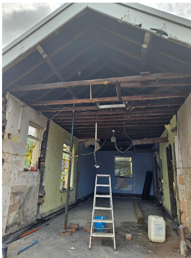
Figure 3 - The house showing external walls and ceilings being removed.
