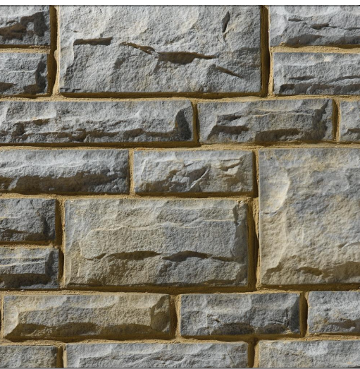
2 Bradstone Square dressed stonework
