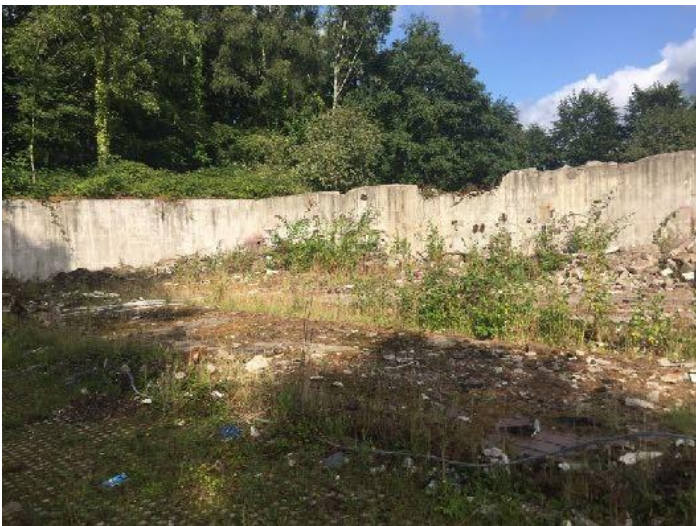
View of building foundations
