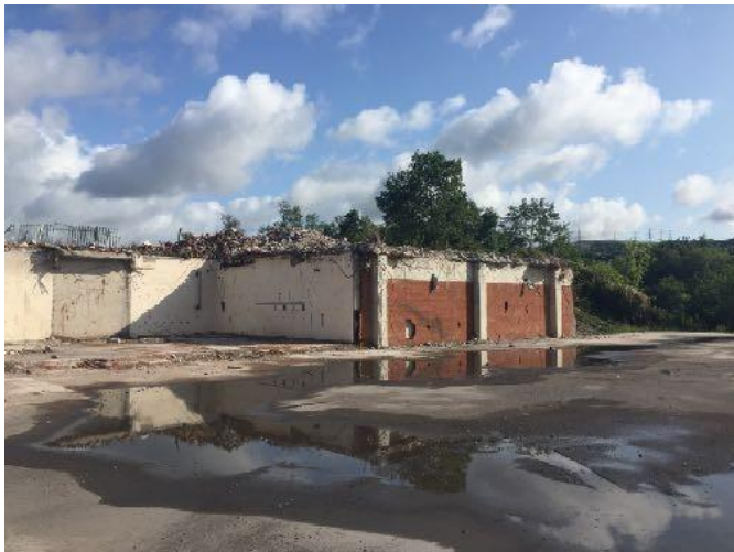
Demolished section of buildings to south of site
