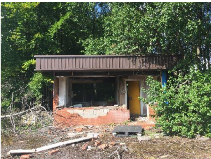
Remaining small building
