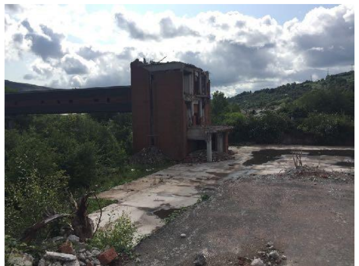
View of south east corner of site
