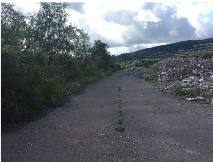
Tarmac road along north east looking south
