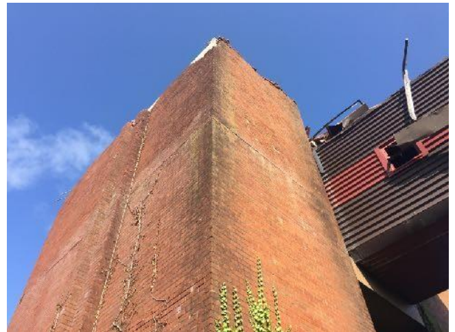
View of Office tower remaining
