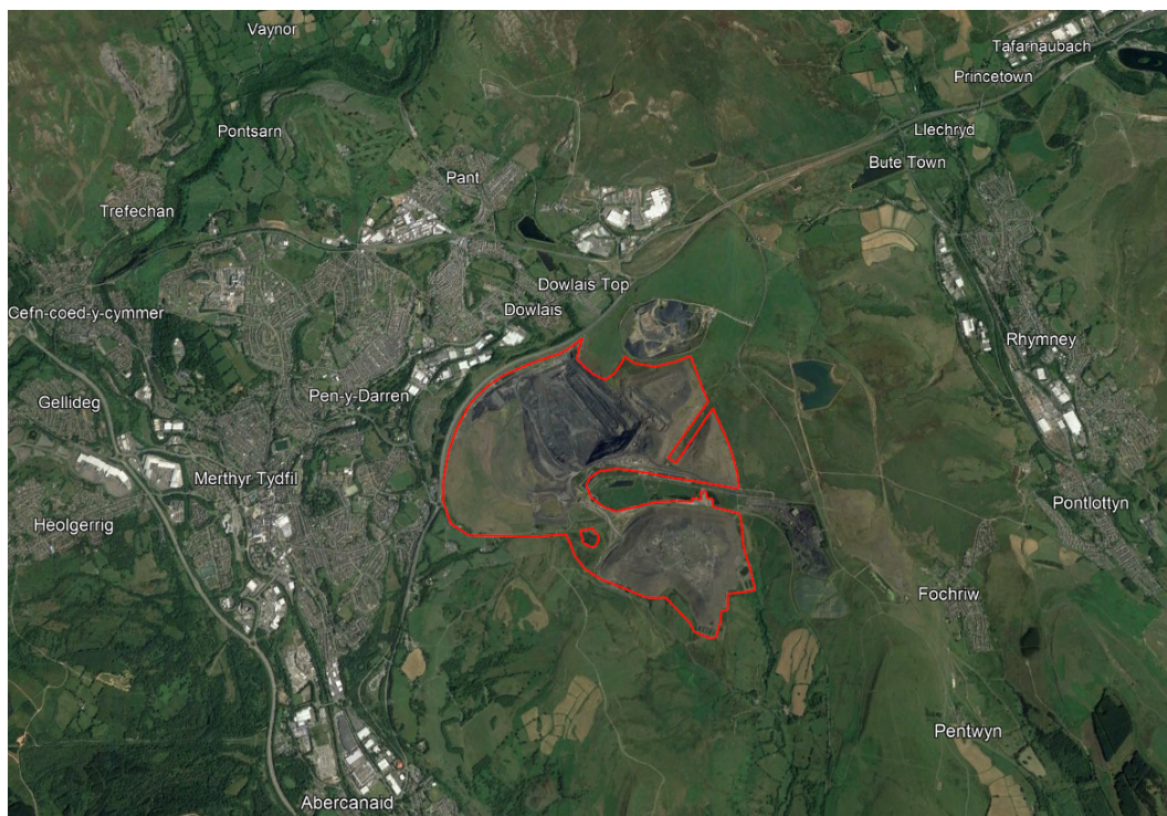
Figure 1: Ffos-y-Fran and Wider Site Setting (Aerial Image)
