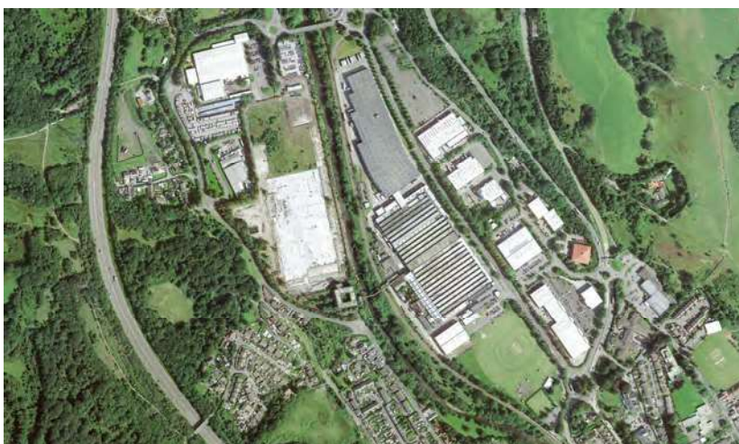
Aerial view of plan showing single redundant Hoover building © Google Earth 2016
