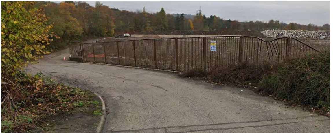
View along recently constructed drainage channel (western boundary)
