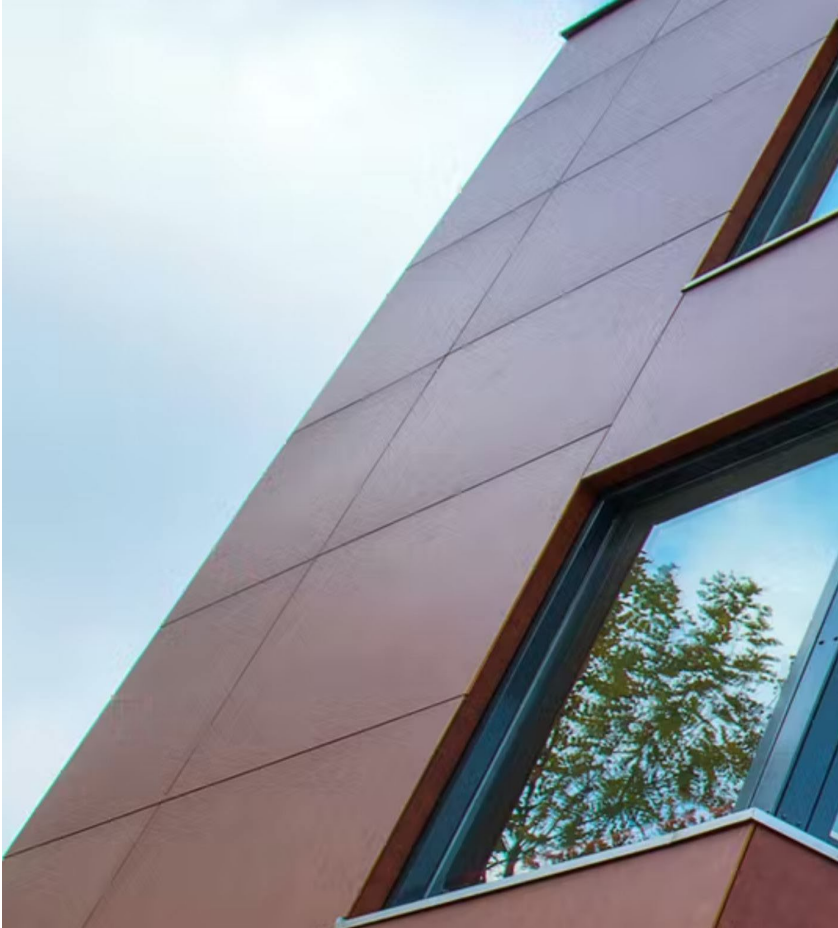
Elevation of Rockpanel cladding – Mineral Rust colour.
