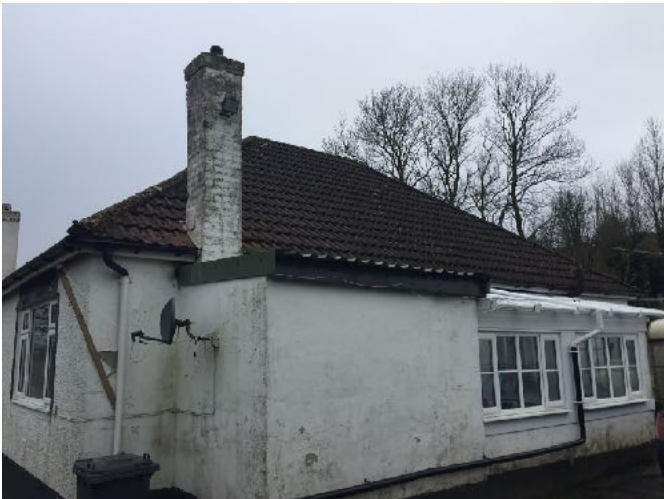
Eastern (rear) elevation of the building
