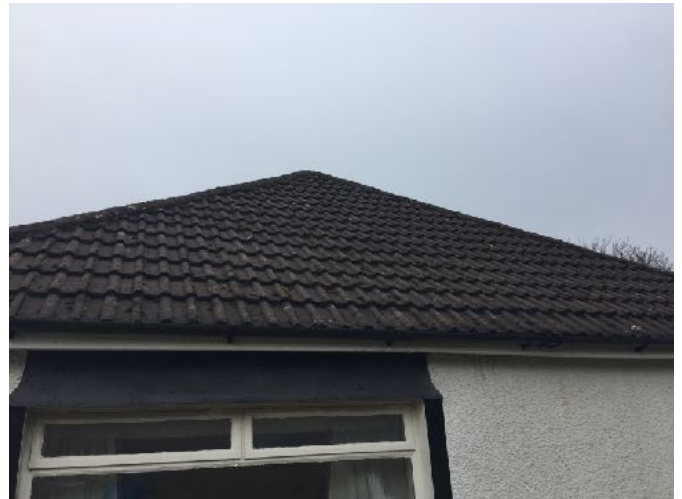
Northern elevation of building
