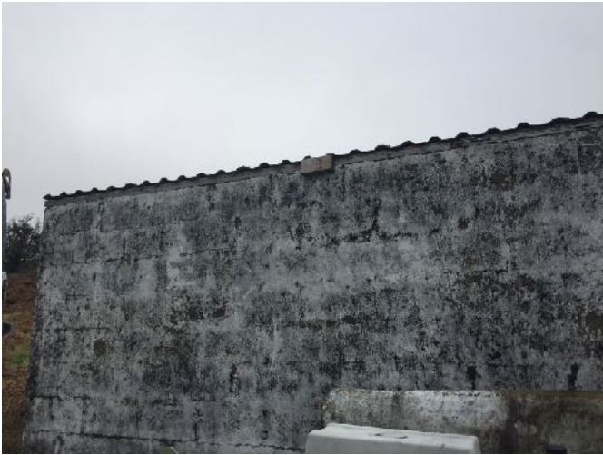
View of outbuilding roof line
