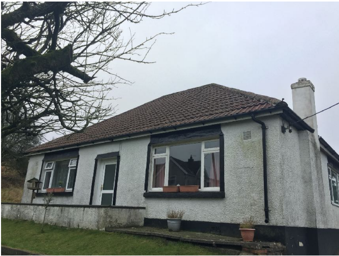
Western (front) elevation of building
