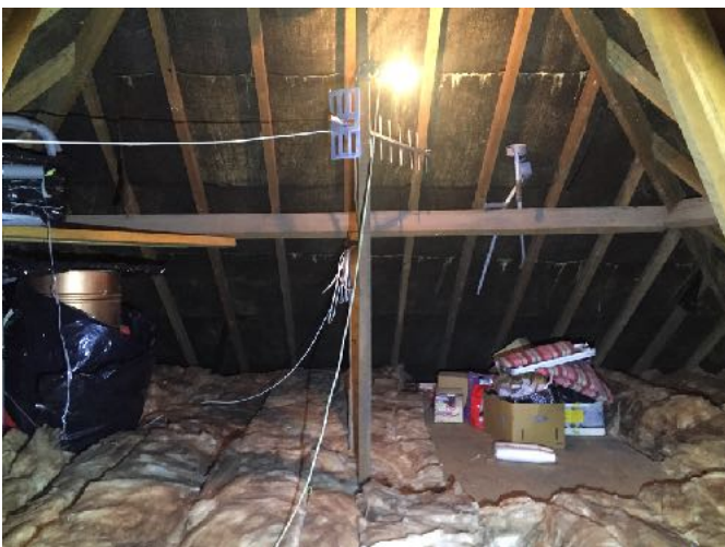
View of attic space
