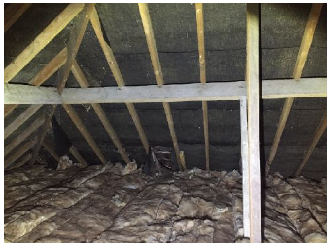
View of attic space
