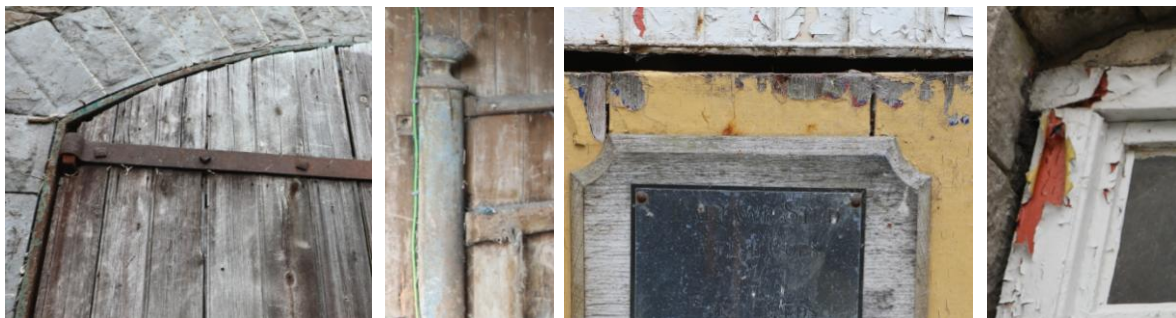
Left to right – green door lining on the Coach House with red (possibly red oxide primer) on its historic ironwork, grey/green on the historic stable stalls, the modern yellow paint on doors over red and, under the red, blue - and white over yellow, red and blue on a doorframe.
