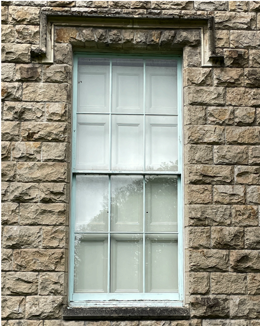
Photo showing the paint colour of the existing windows at Cyfartha Castle
