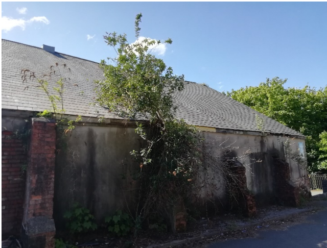
Figure 10 - North western aspect of the building
