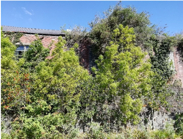
Figure 6 - Southern aspect of the building
