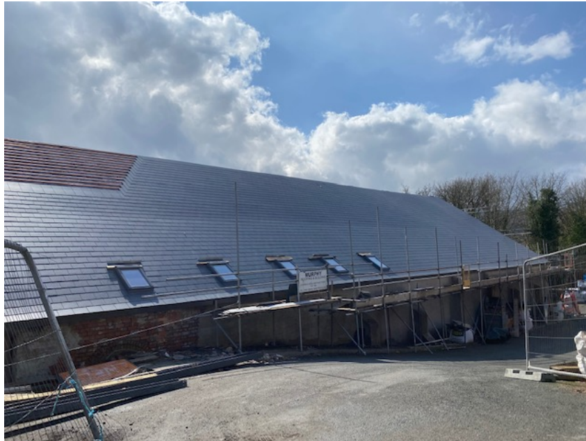
Figure 4 – northern elevation showing new roof covering (provided by client)
