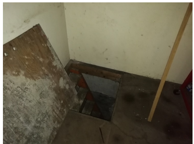
Figure 15 - View of basement store access
