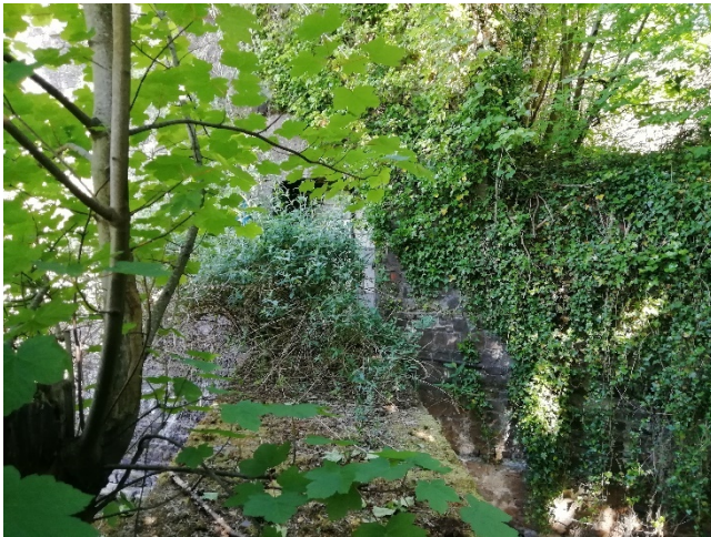
Figure 8 - Dense ivy growing on the building
