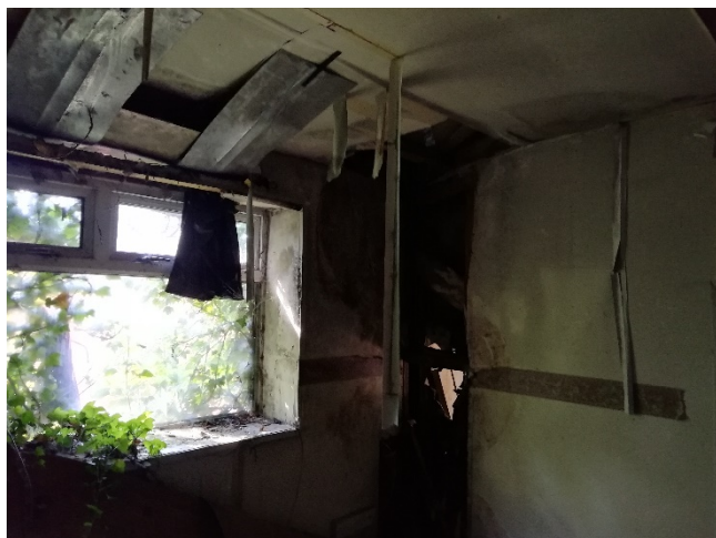
Figure 16 – Upper floor office room (window to southern elevation)
