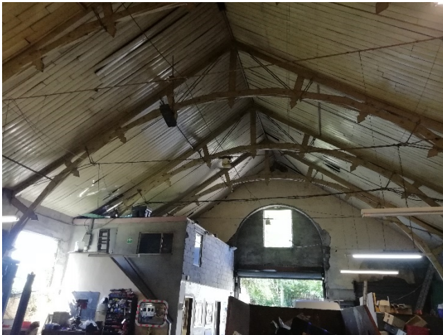
Figure 12 - Inside workshop showing wooden beam roof structure
