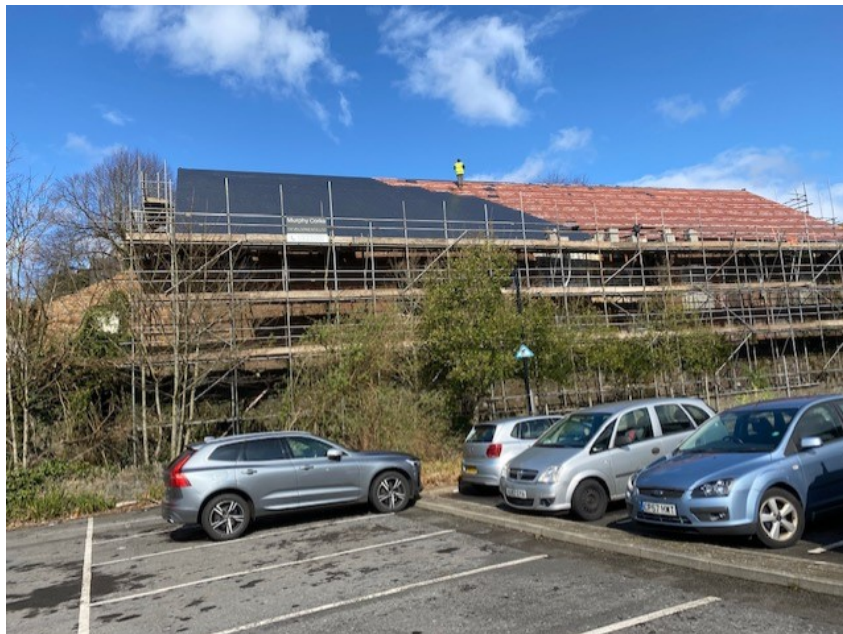
Figure 5 - southern elevation showing new roof covering (provided by client)
