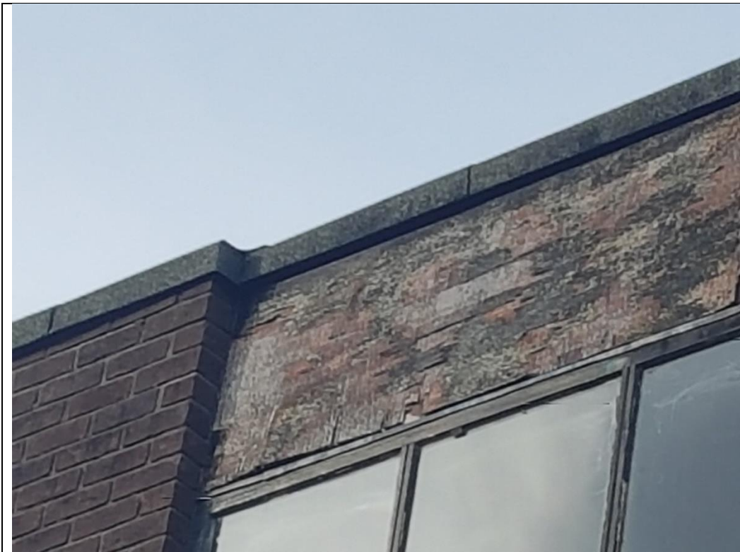
Photo 5. Gaps in boarding to east
