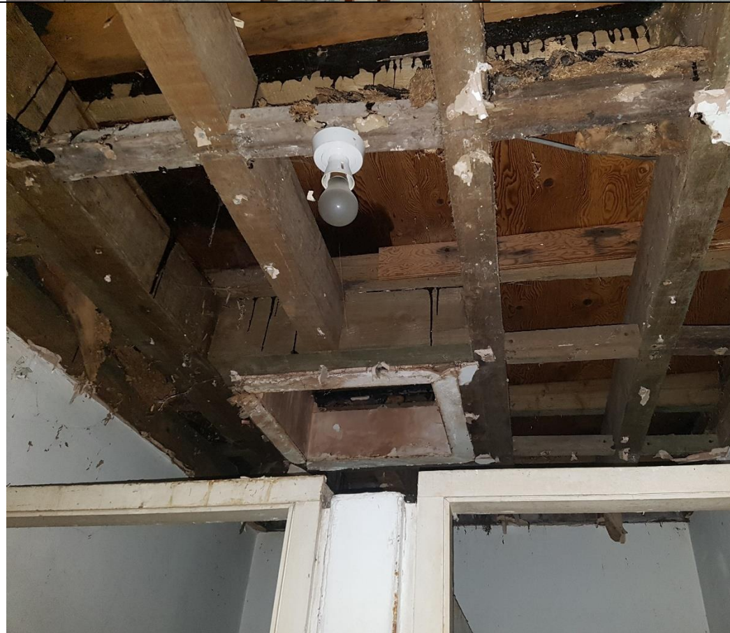
Photo 10. Ceilings removed in the toilets
