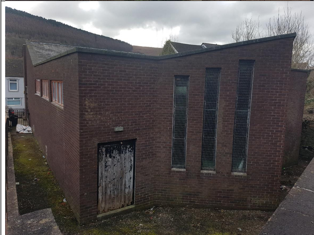
Photo 2. Side (north) elevation and part of west
