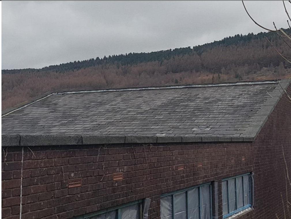
Photo 8 Slate mono- pitch with some misalign ed sltes
