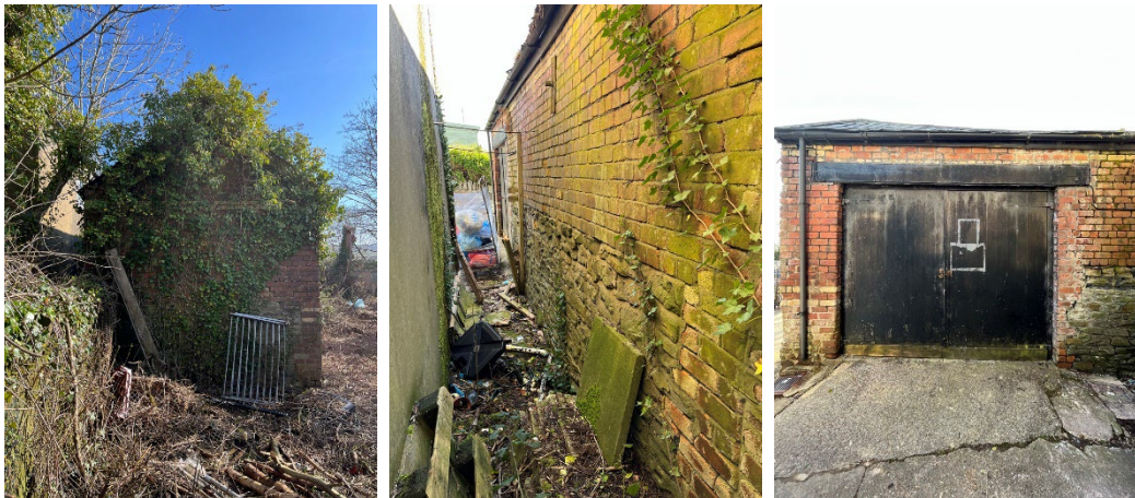
Photo 3: Southwest view of the gable end; Photo 4: Northeast view of the side elevation. Photo 5: Facing view of the large double door entrance.
