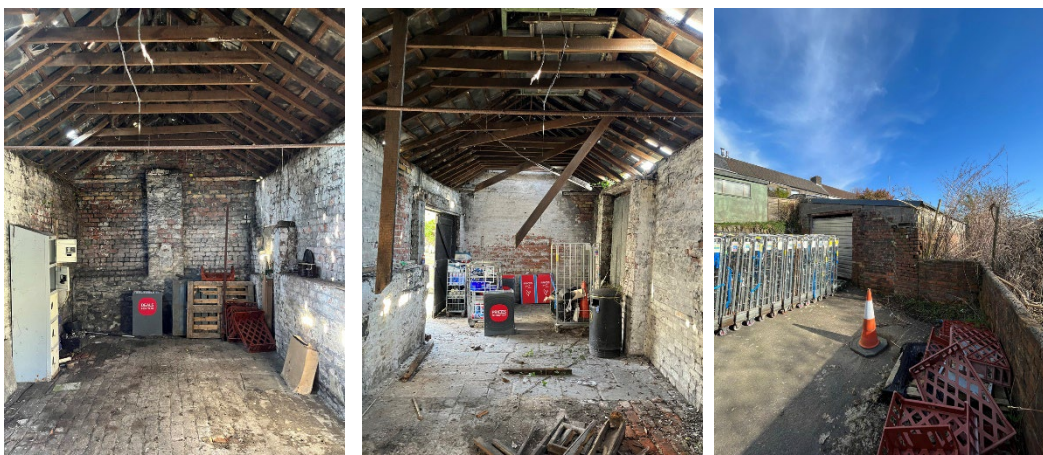
Photo 6: Internal view facing southwest; Photo 7: Internal view facing northeast; Photo 8: Further outbuilding which appears on the same OS map.
